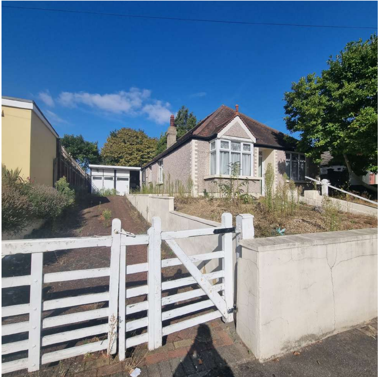
Image looking at the front of 108 Havelock Road.
