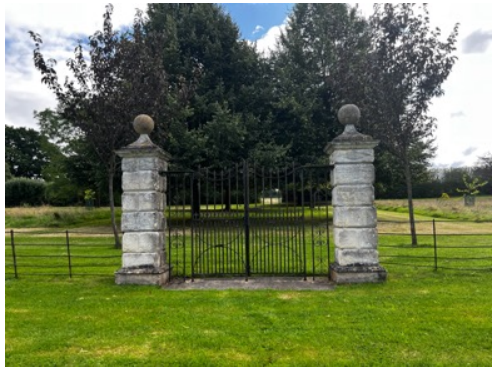
Existing gates to west of the property
