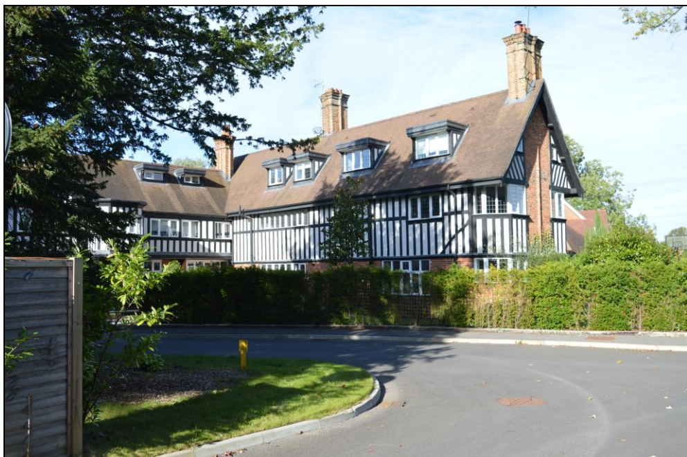
Winchfield Lodge has been converted by reason of the 2013 application and forms a central feature of the housing cluster
