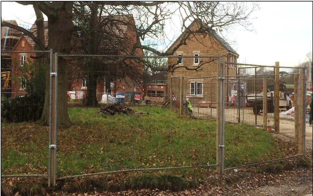
Weld-mesh panels on wooden posts
