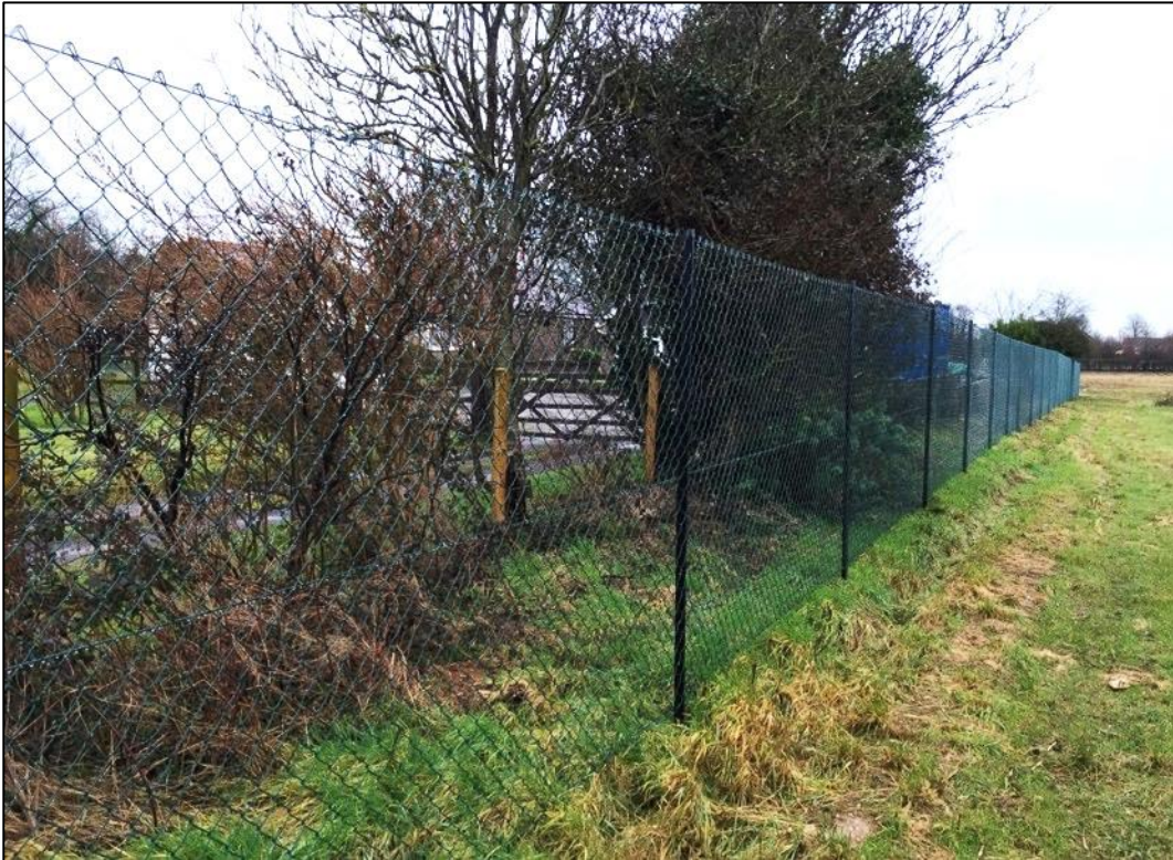
Chain-link on angle-iron uprights
