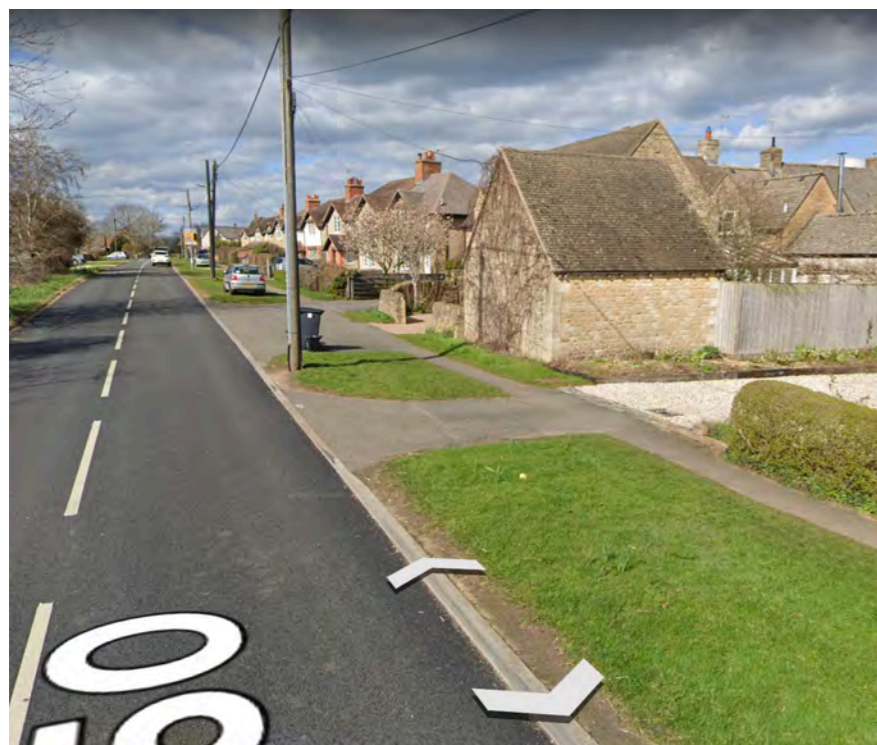
View of south and west elevations of the garage
