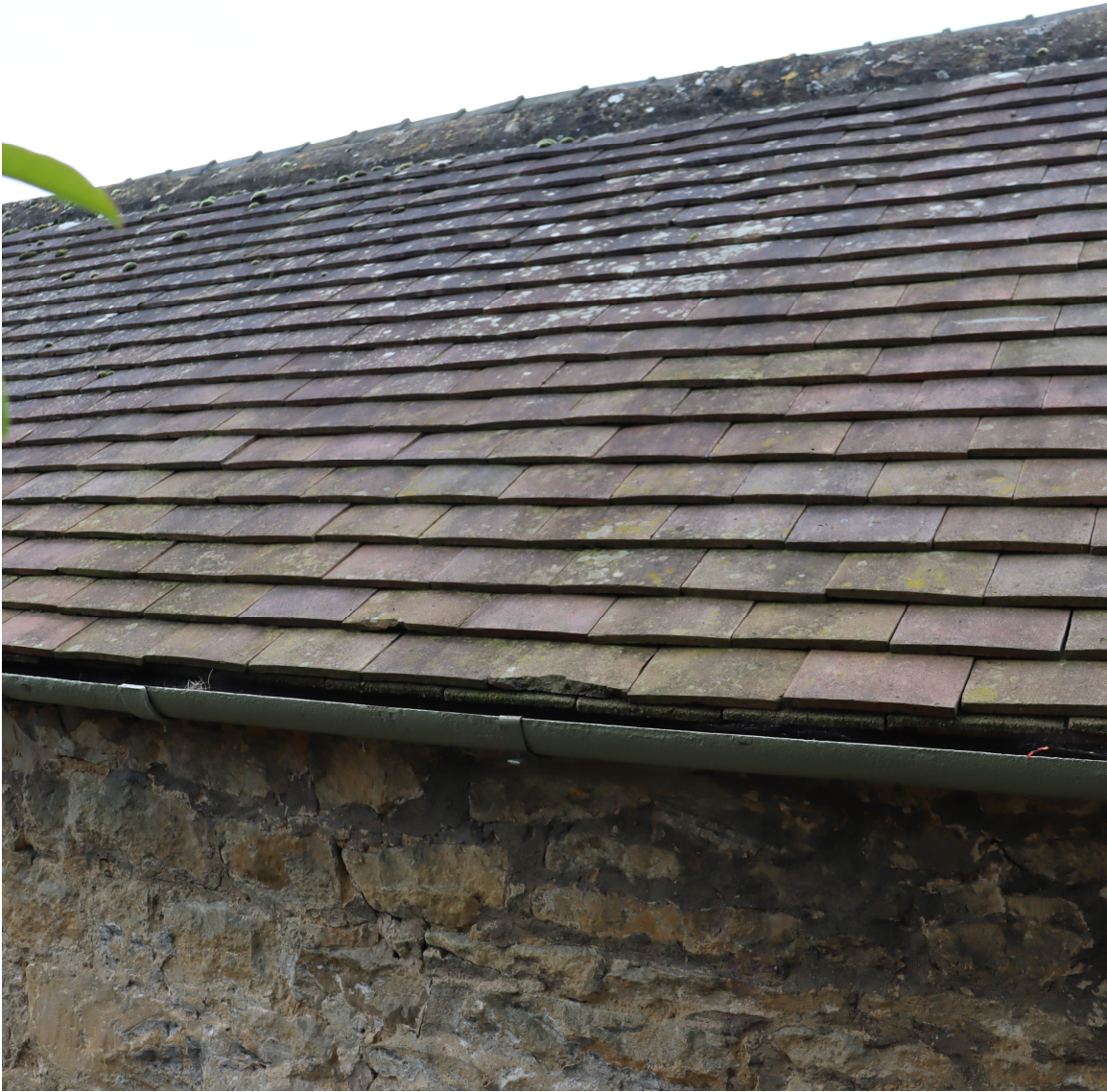
Re-claimed tile roof finish showing cast iron gutter
