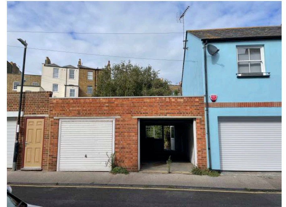
IMAGE 01 View of existing Telford St elevation
