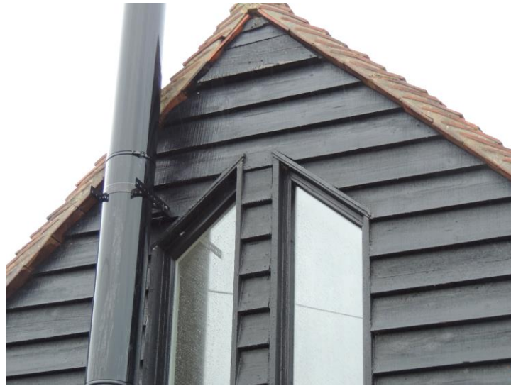
Photo 7: Note tight seal to gable
