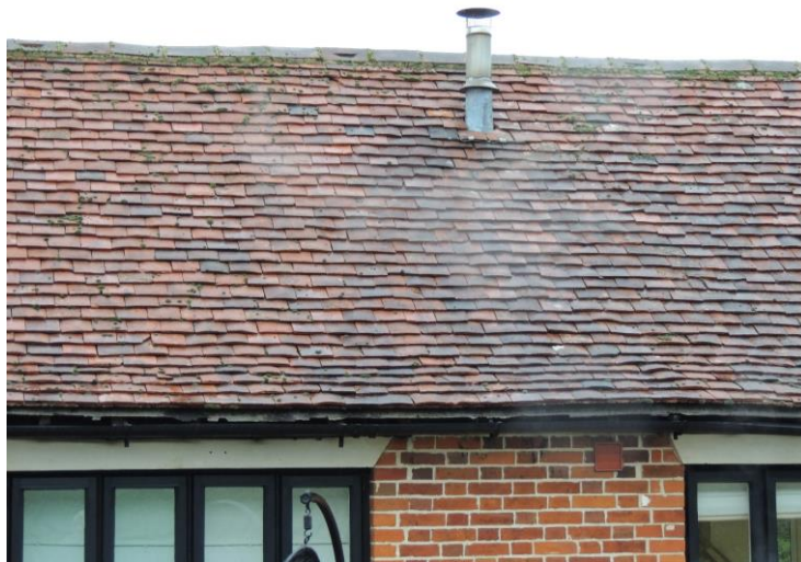
Photo 10: Note tight seal to roof tiles
