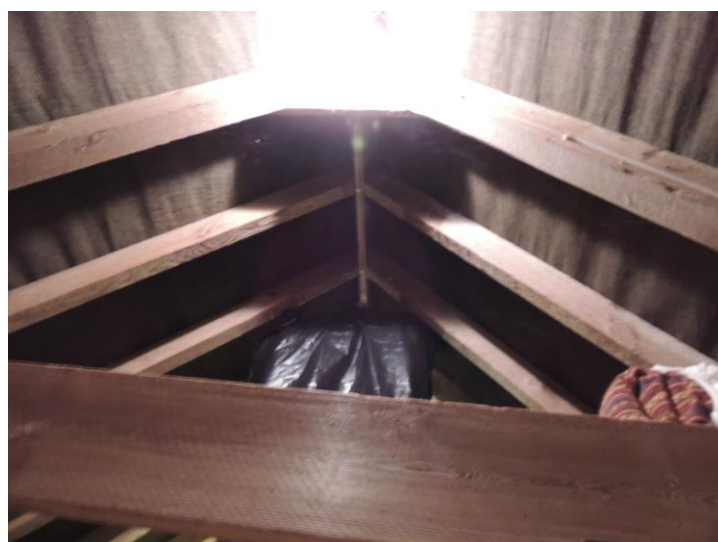
Photo 6: The roof had no features that might be occupied by bats
