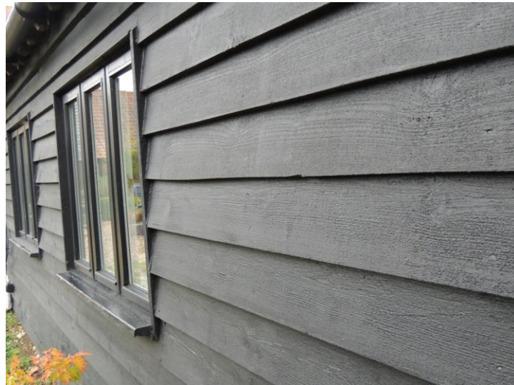
Photo 8: Note tight seal to cladding
