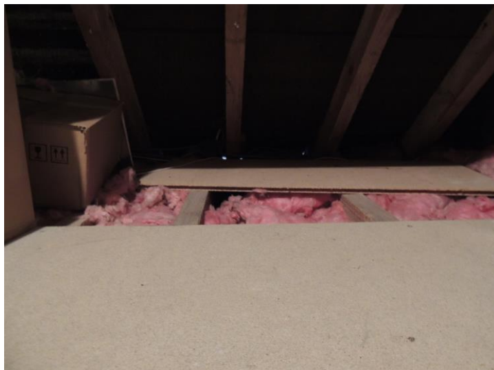
Photo 4: Note lack of evidence of bats on boarded floor
