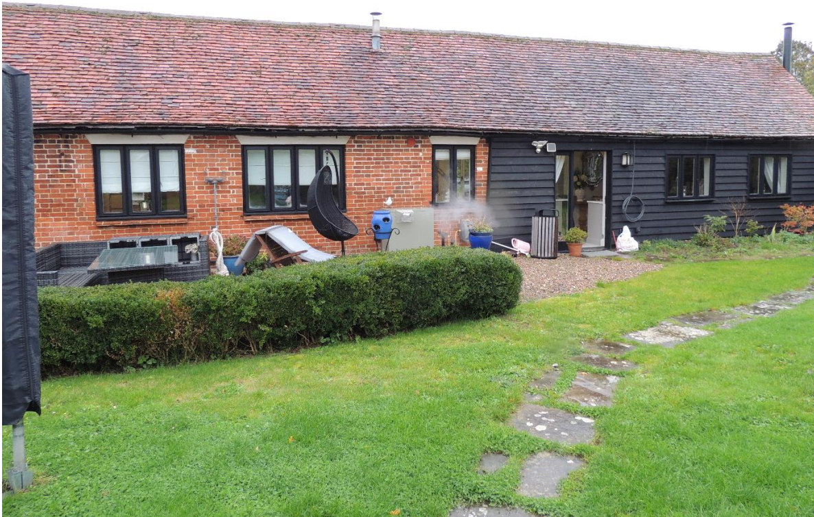
Photo 1: Western elevation. The proposal is for two extensions on this side of the property
