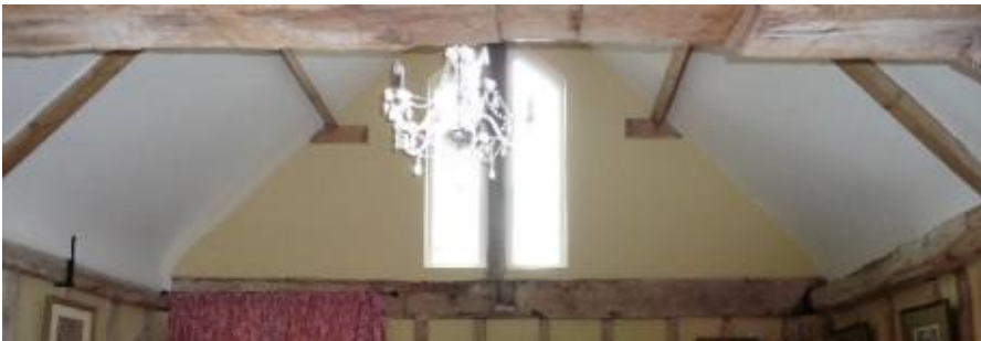
S wall plates and modern side purlins roof above
