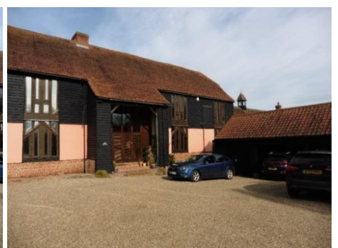
South façade east end
