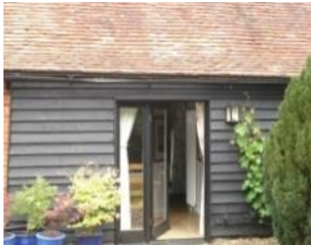
West façade – retained doorway
