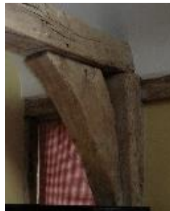
tie beam& braces
