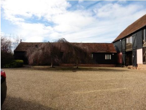
SW range east facade
