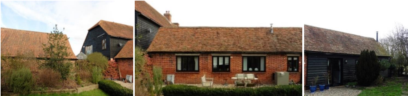
Outbuilding & Barn West facade
