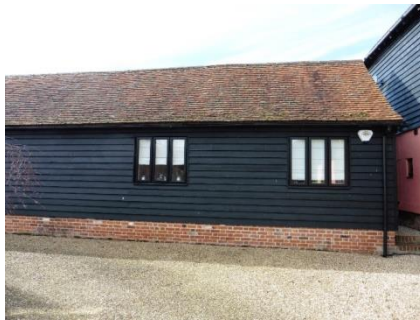
SW range east façade north end
