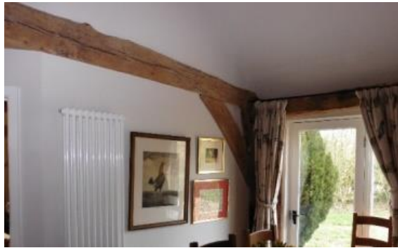
Tie beam, brace & doorway
