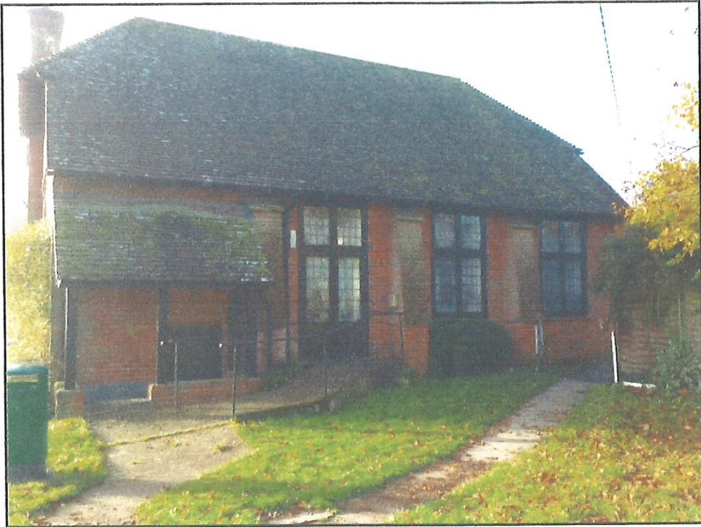
Side of club, north facing, no change.
