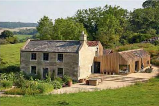
Modern single storey extension to existing old structure. Natural materials help blend the extension into site and compliment existing building and surroundings. Modern extension set back from site frontage to make it subservient.
