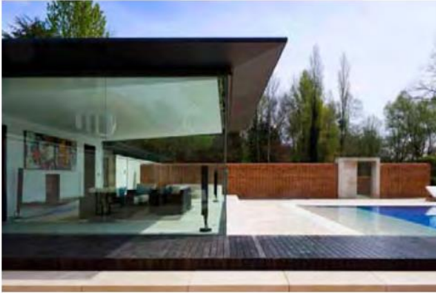
Use of minimal glass framing and slim overhangs to give the impression of a cantilevered/floating ceiling.
