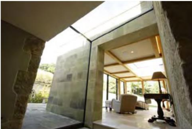
Minimal framed glazed link between two spaces. Creates very airy connection space and allows interaction to outside.
