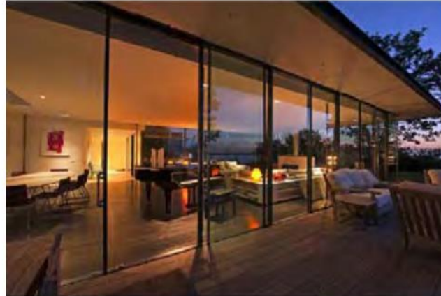
Over sailing glass with large overhangs to help with solar shading and the effect of a floating ceiling
