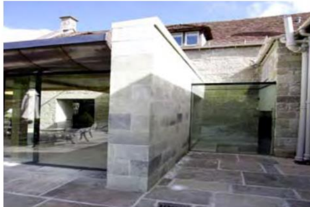
External view showing juxtaposition of existing stonework, old traditional features and new contemporary glazing.
