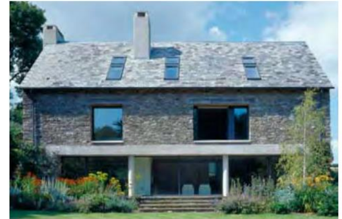
Use of modern minimal framed glass on a traditional style building. Use of skylights carefully placed to align with elevations below.
