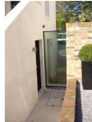
Glass link showing new connection to existing older spaces.
