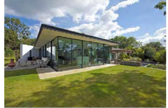
Glass over sailing ceiling thickness to give the impression of a thinner ceiling creating a lighter feeling to the building.
