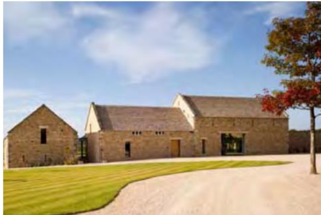
Conversion of existing buildings with modern architectural additions/finishes and landscaping to create a more contemporary setting. Use of minimal framed transparent glazing so as not to subtract from buildings original form
