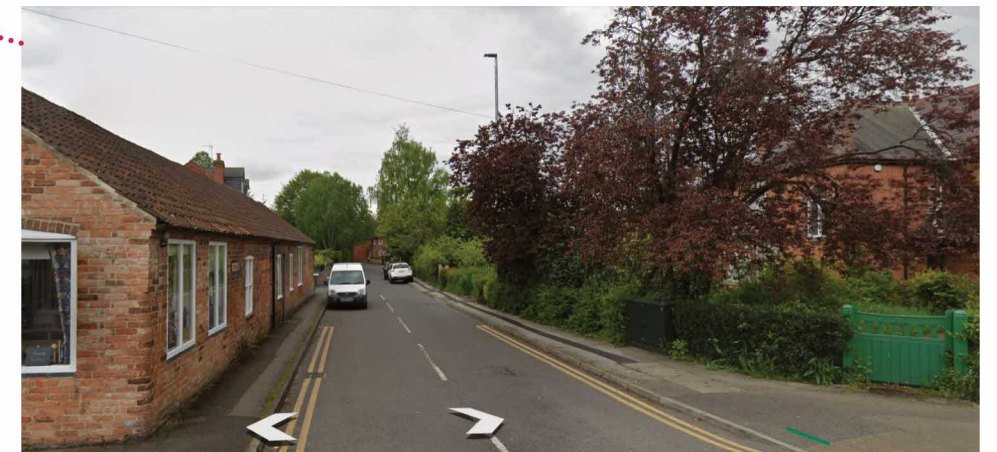
Junction between Main Street and Ton Lane, relationship between Grade II listed building and proposed site
