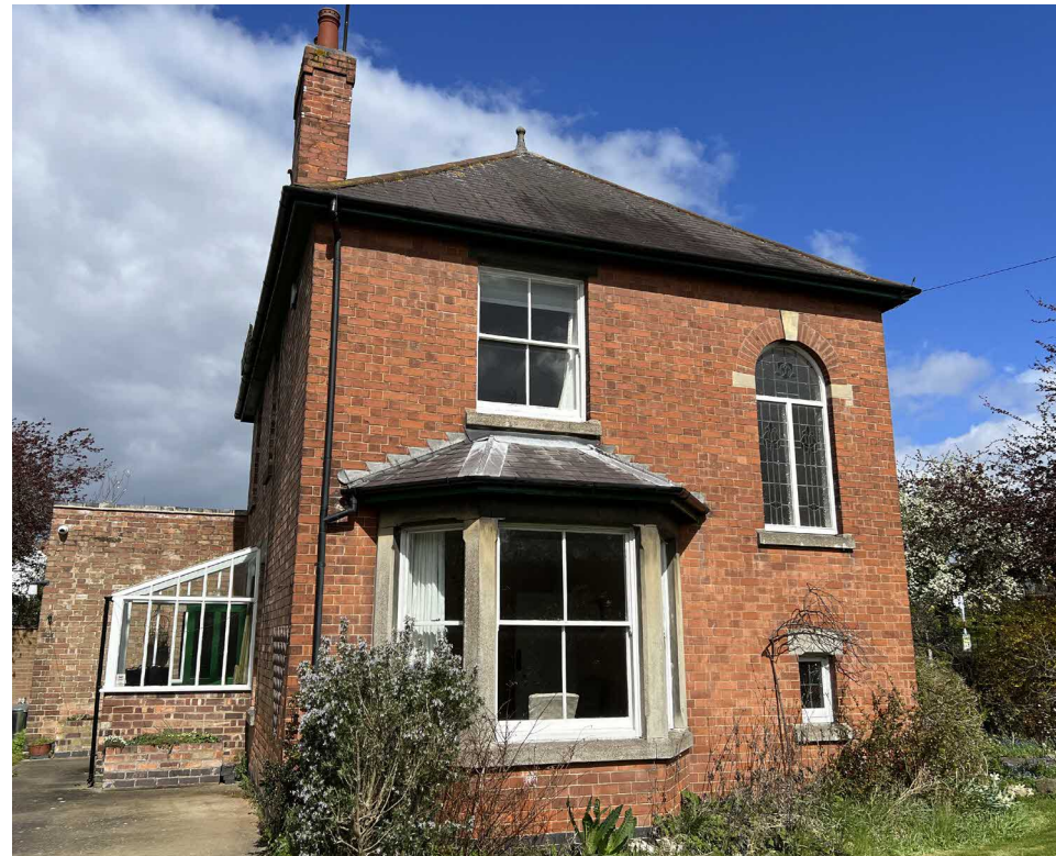
Existing Elevation to Ton Lane
