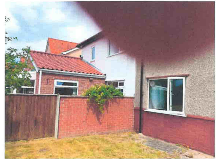
Rear view showing existing rear / side extension to neighbouring property. Proposed development shows symmetry to this design.
