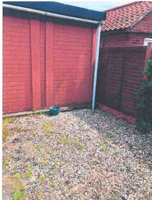
Border fence to be retained and repaired as necessary
