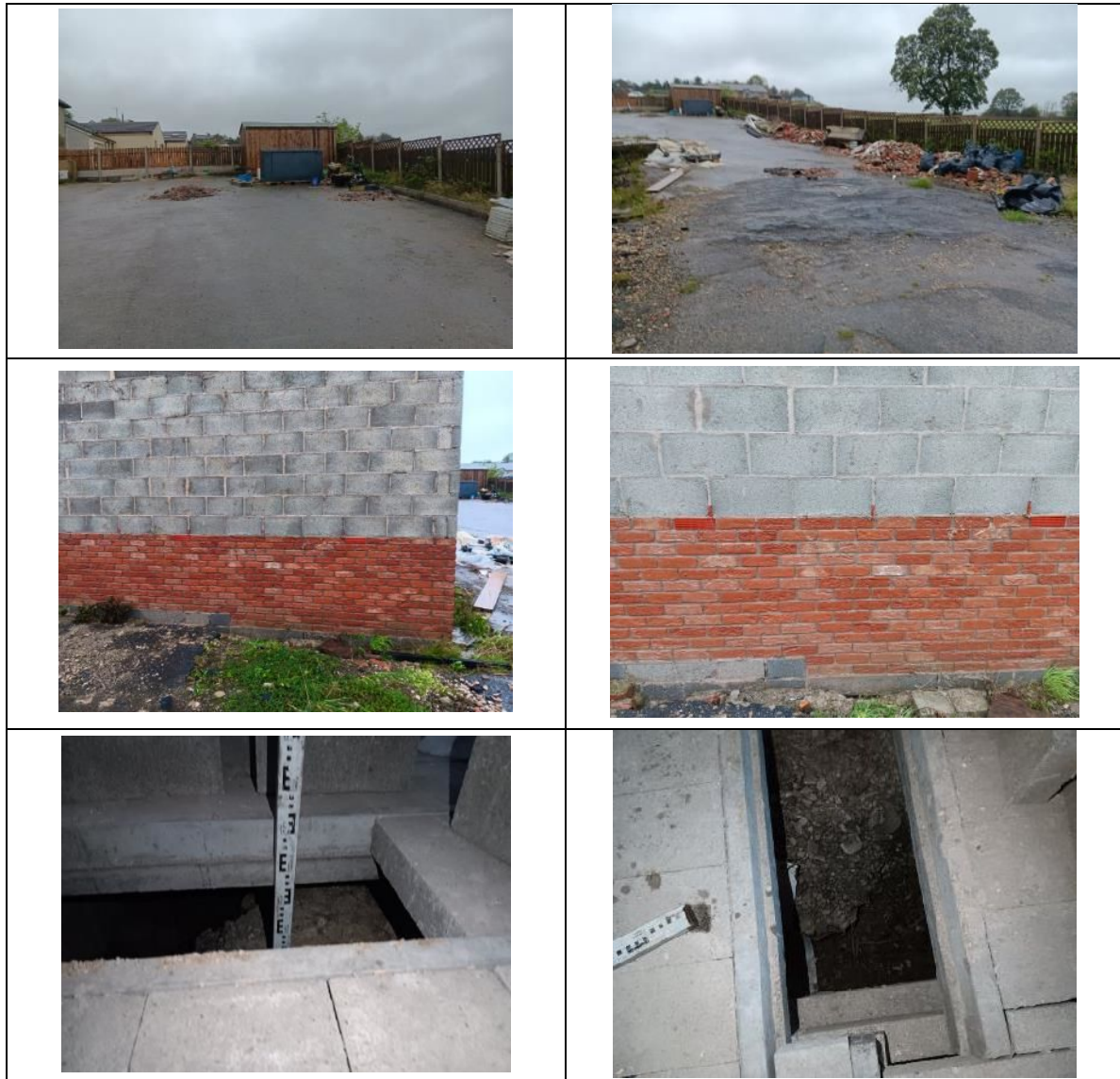
Plate 2-1: Site visit photos
