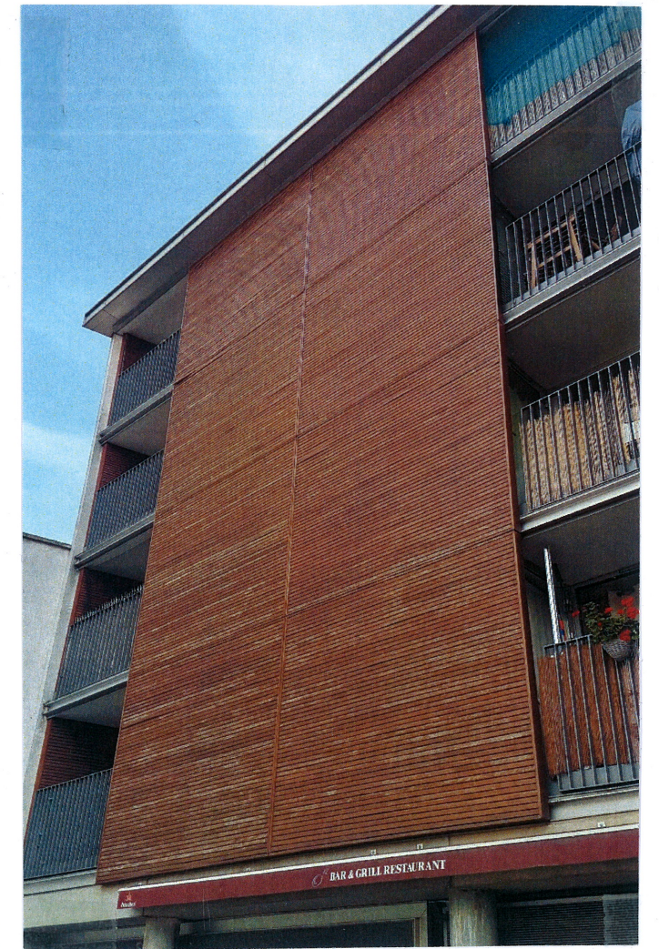
photograph rear elevation (typical timber cladding)
