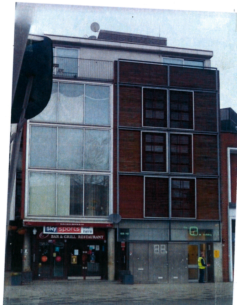
photograph front elevation (timber cladding panels)
