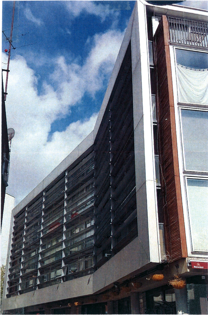
photograph side elevation (timber clad panels on corners)
