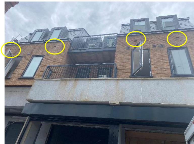
Figure 3 x4 swift nest boxes in the brick work (circled).
