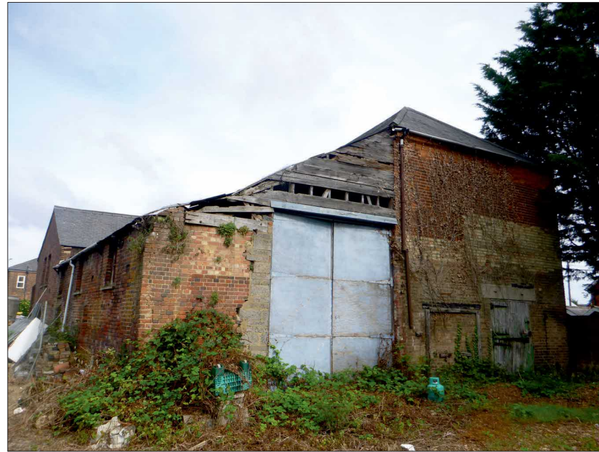
Photograph 2: Showing the rear of the Warehouse (B1).
