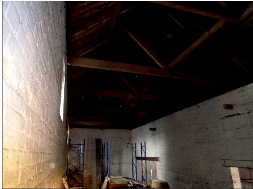
Photograph 5: Showing the vaulted roof of the Warehouse (B1).
