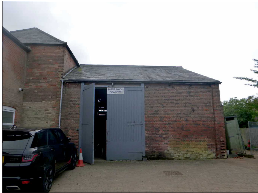
Photograph 1: Showing the front of the Warehouse (B1) and associated hardstanding.
