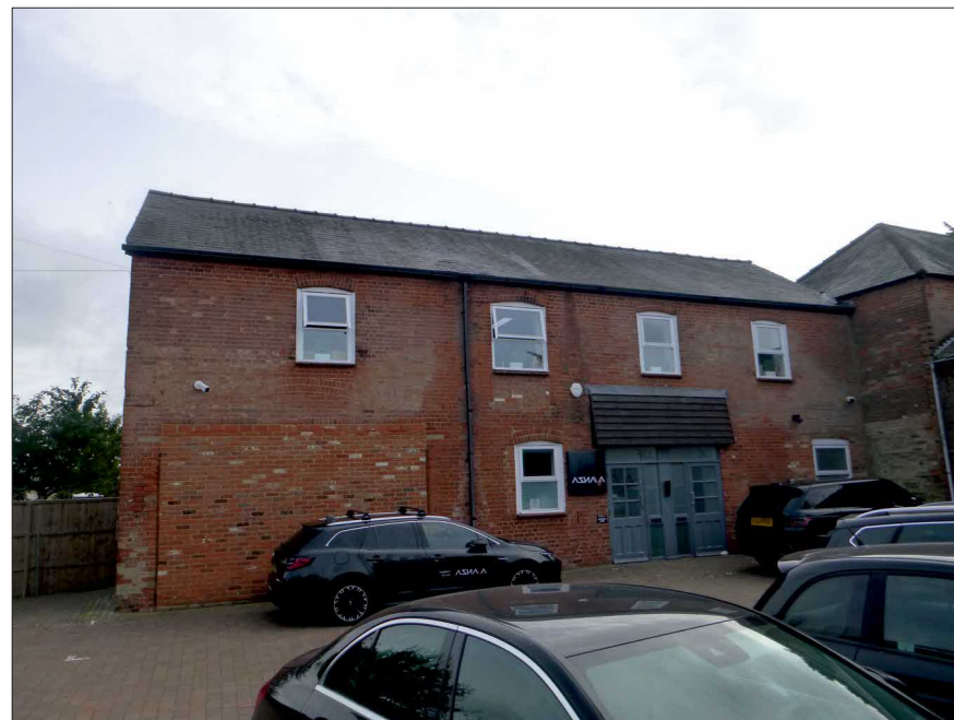
Photograph 4: Showing the front of the Western Office (B4) and associated hardstanding.
