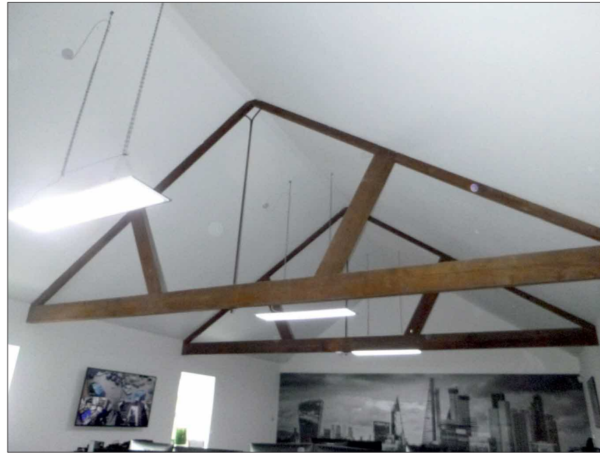
Photograph 6: Showing the vaulted ceiling inside the Western Office (B4).
