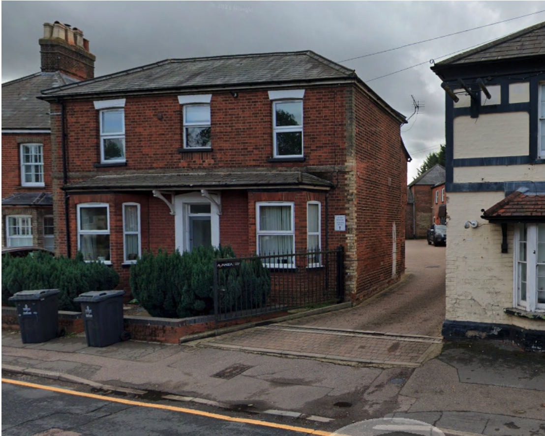
View of front of 33 Julians Road (to be retained)
