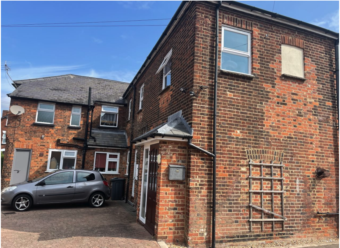
View of rear of 33 Julians Road (to be retained)
