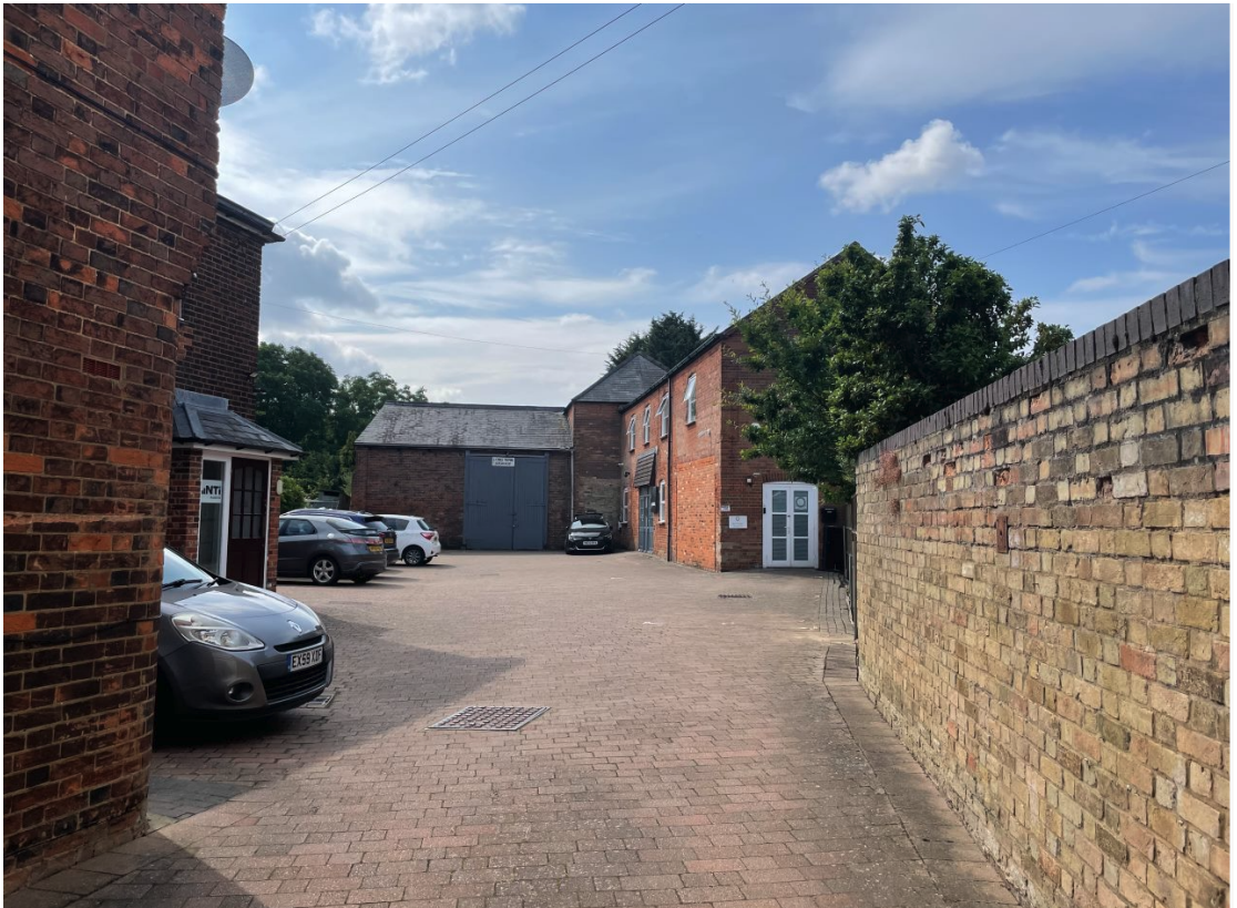
Existing view of the 'yard buildings' from the entrance off Julians Road
