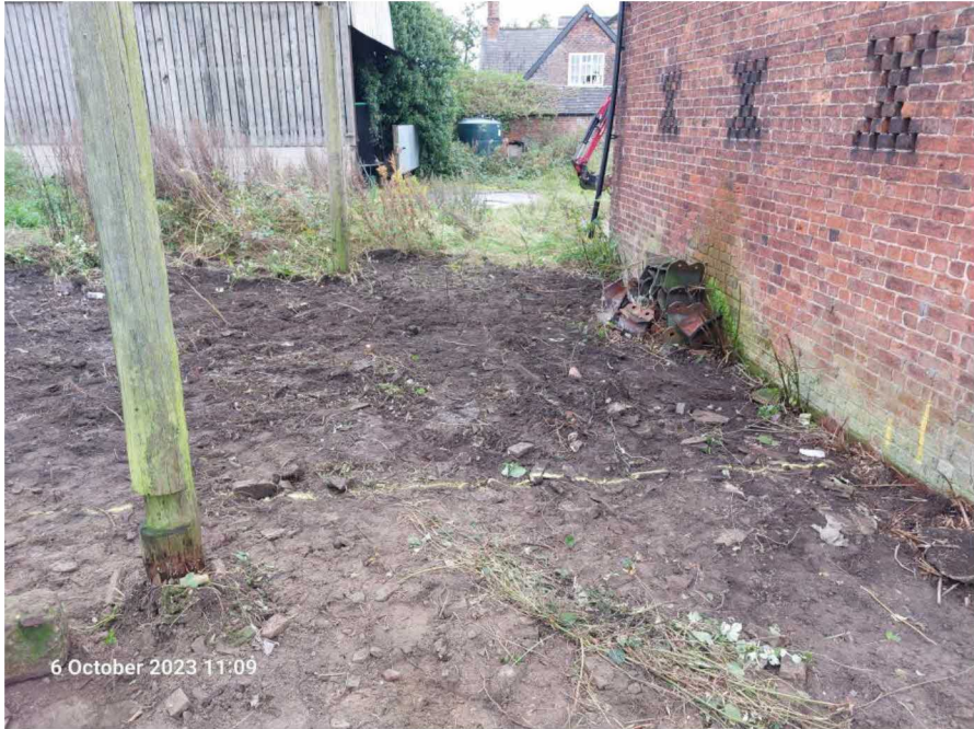
Figure 7 – Showing the removal of vegetation behind the Coach House.
