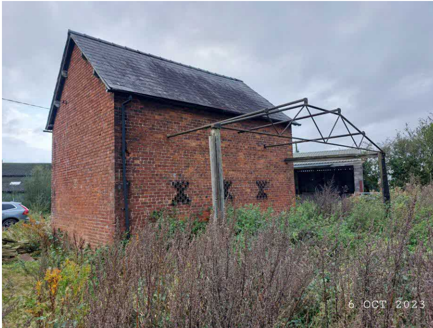
Photo 2 – Showing the Coach House before commencement began on the 6 th of October 2023.
