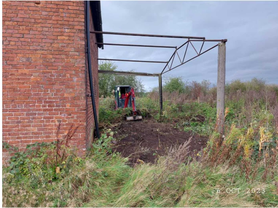
Figure 6 – The site during the commencement works.
