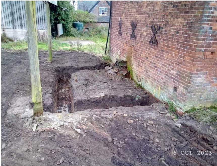
Figure 12 – The dug out footings demonstrating commencement on site at Manor Farm.
