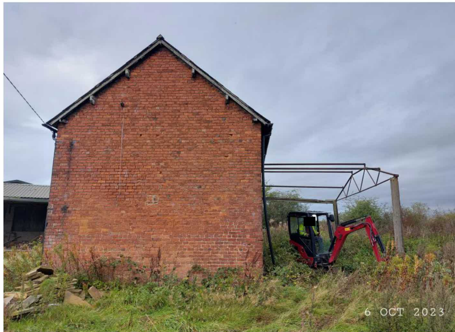
Figure 5 – Photo showing the commencement work taking place at the coach house.
