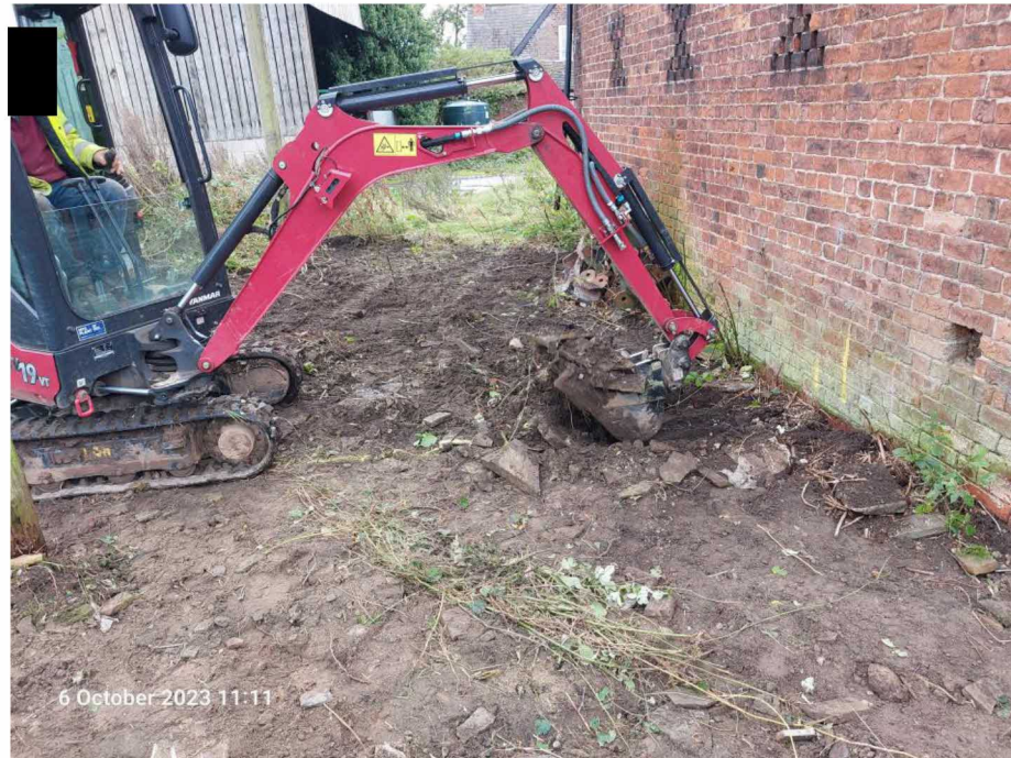
Figure 8 – Showing operations on site to create the footings.
