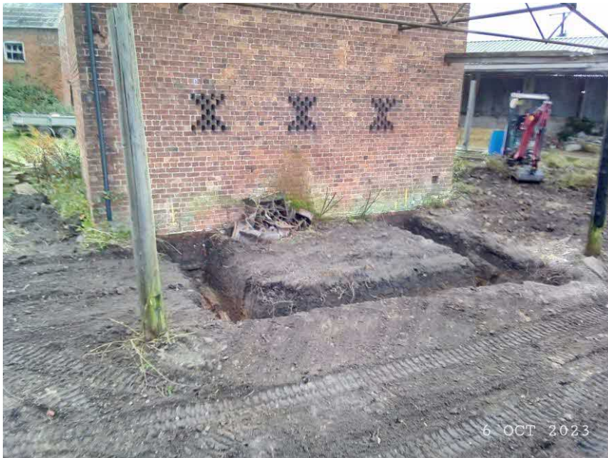
Figure 11 – The footings upon the completion of commencement works at Manor Farm.
