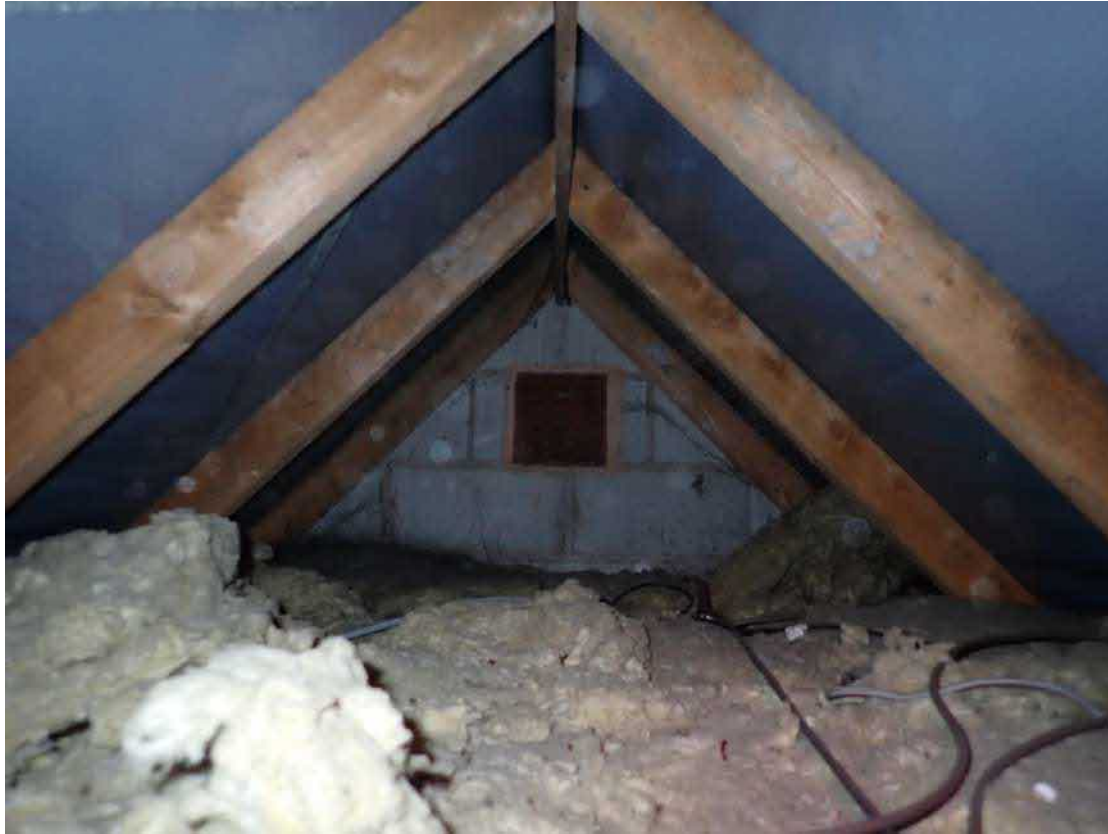
Photograph 9 – looking east to west across the loft space.
