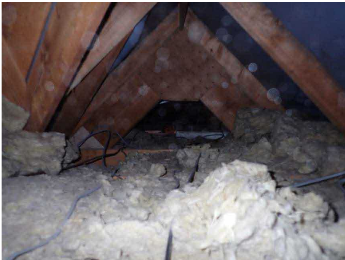
Photograph 10 – looking west to east across the loft space.
