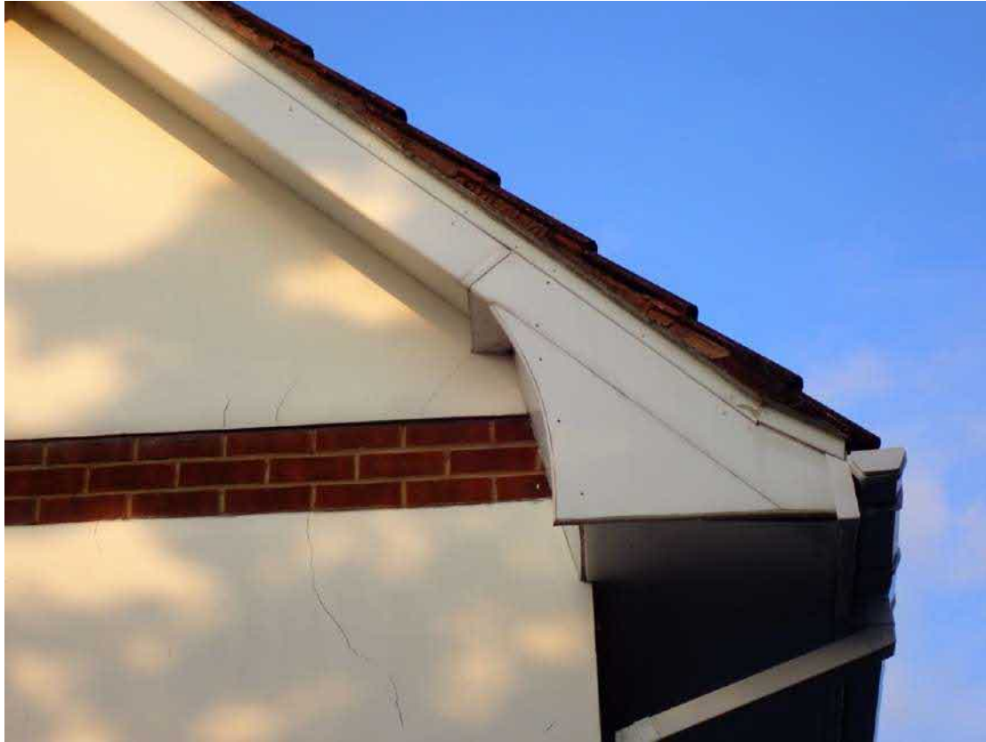
Photograph 7 – plastic box soffits are well maintained.
