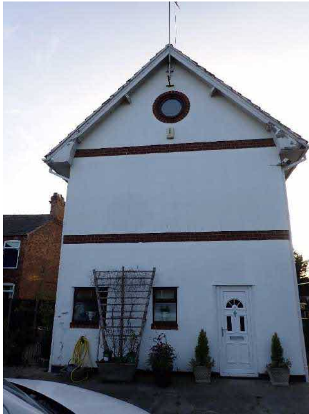
Photograph 3 – eastern aspect of the building.
