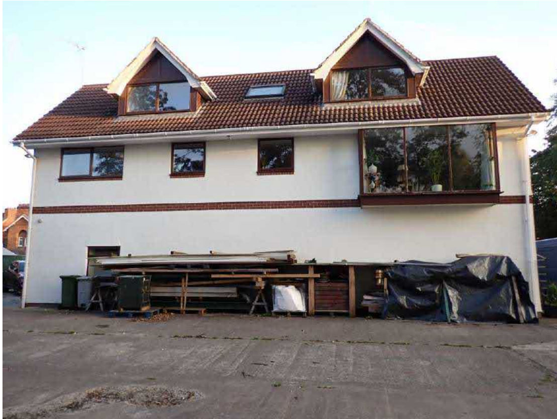
Photograph 1 – northern aspect of the building (rear).
