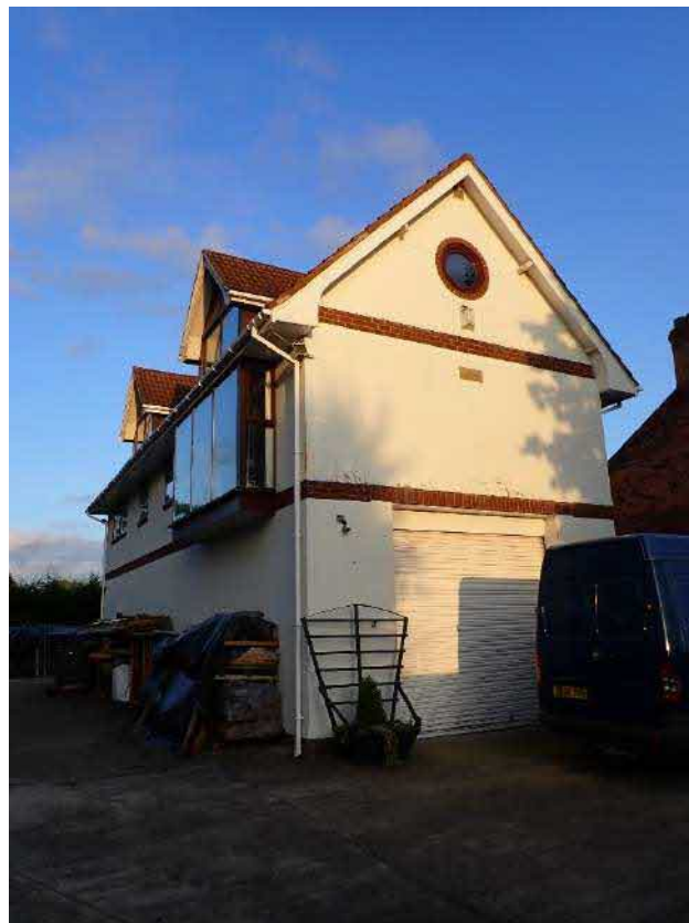
Photograph 4 – west aspect of the building.
