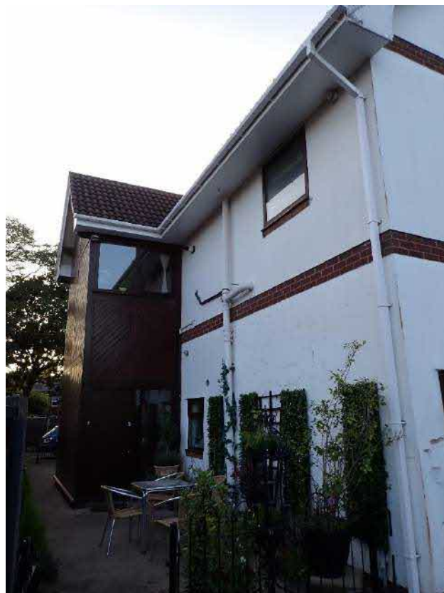
Photograph 2 – southern aspect of the building (front).
