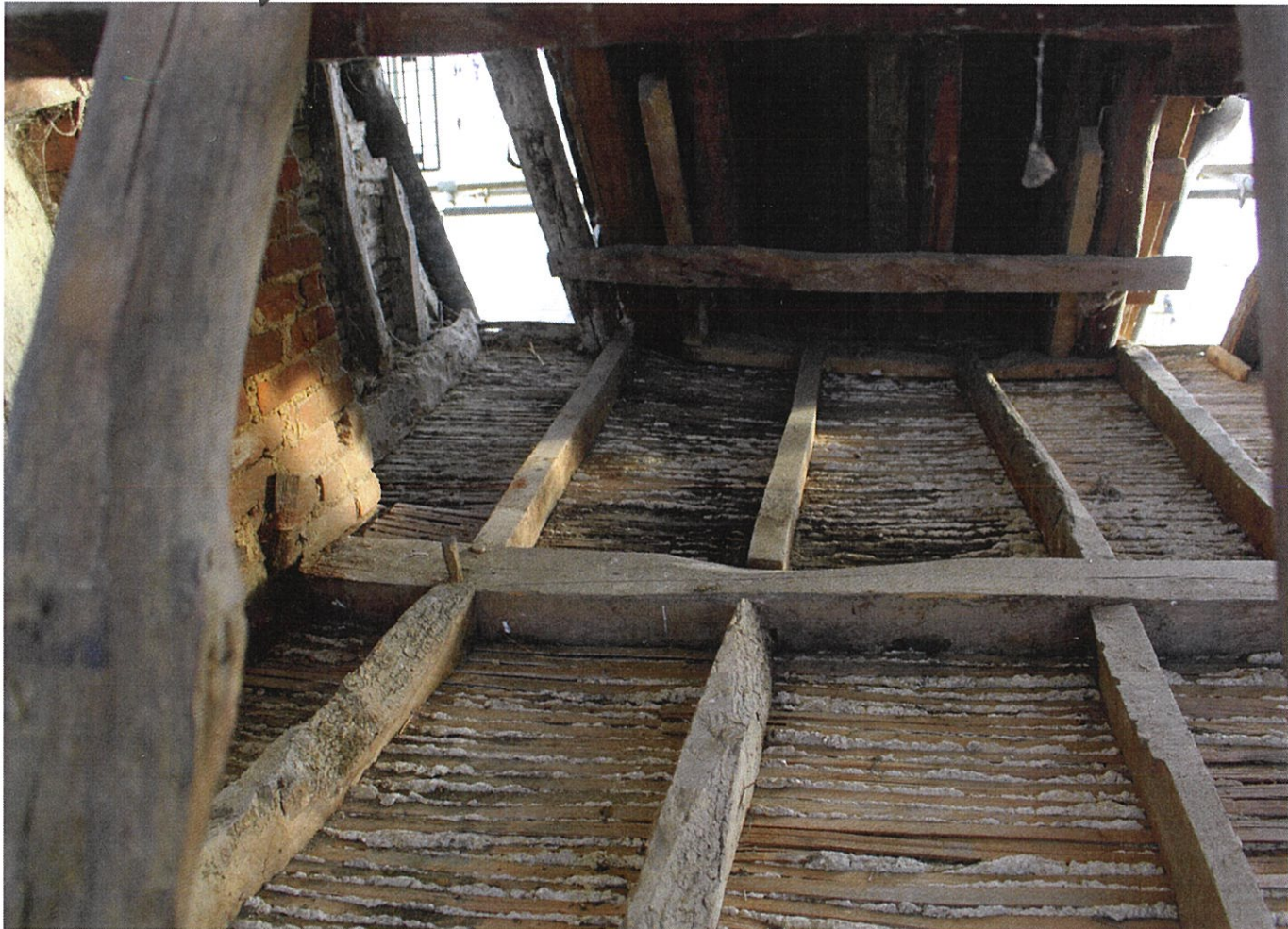
↑ CEILING WHEN SPINE BEAMS IN TWO BAYS ARE CRACKED -
