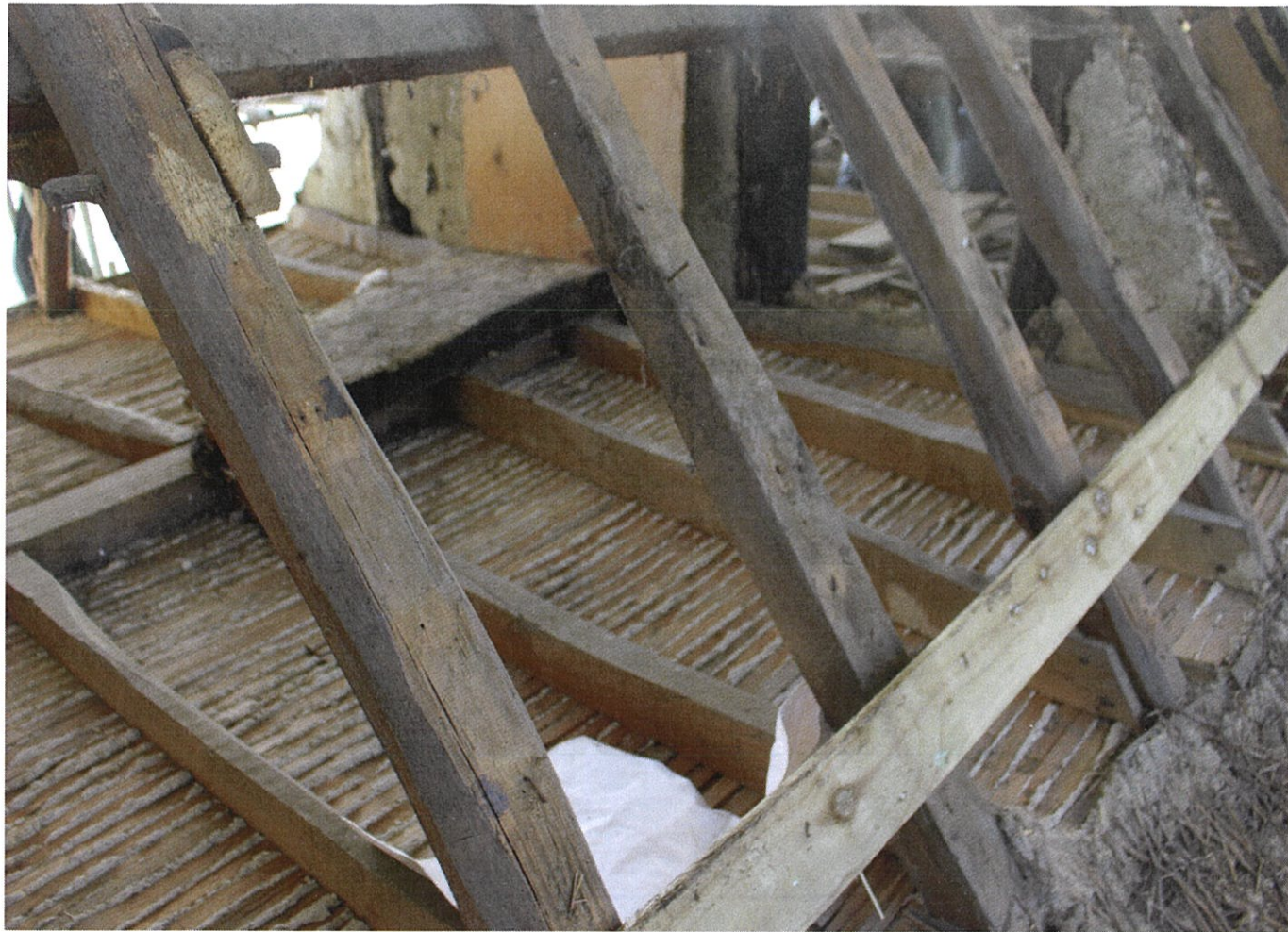
↑ CEILING WHEN SPINE BEAMS IN TWO BAYS ARE CRACKED -
