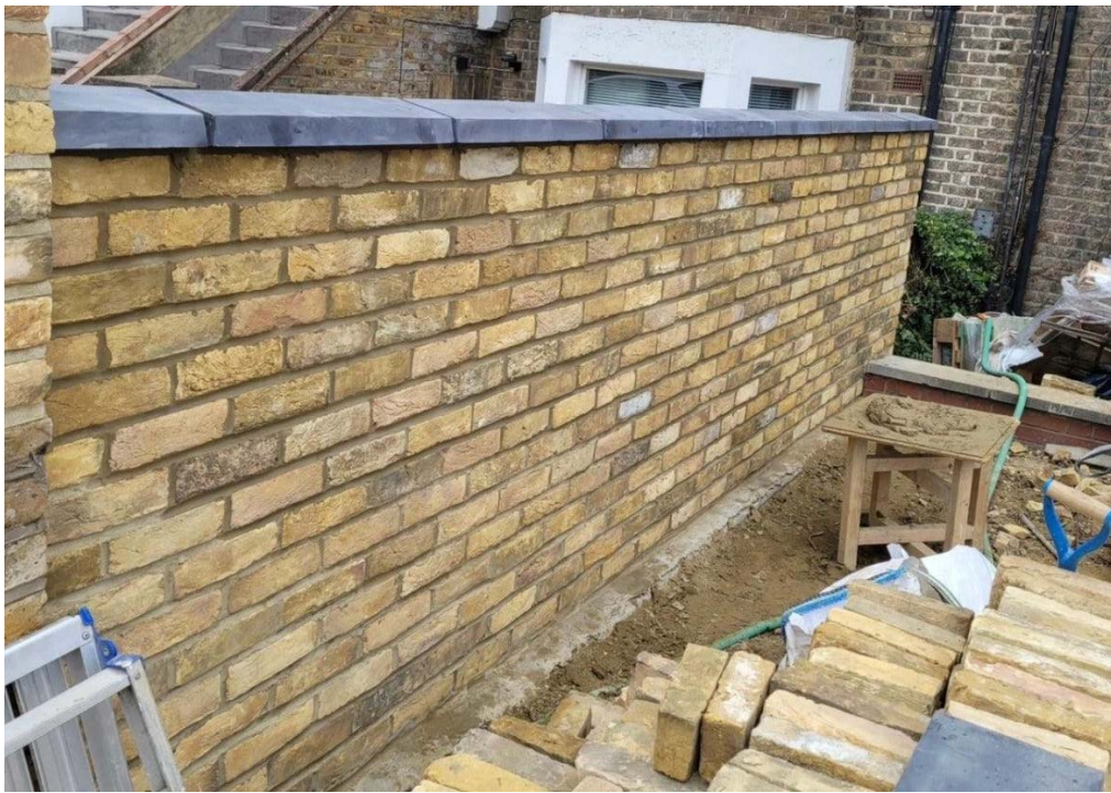
Figure 3 – Built example using London yellow stock brick, image from Reclaimed Brick Company
