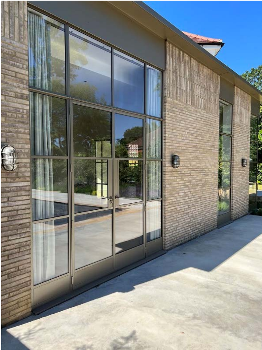
Figure 5 – RAL 1035 glazing set within buff brickwork
