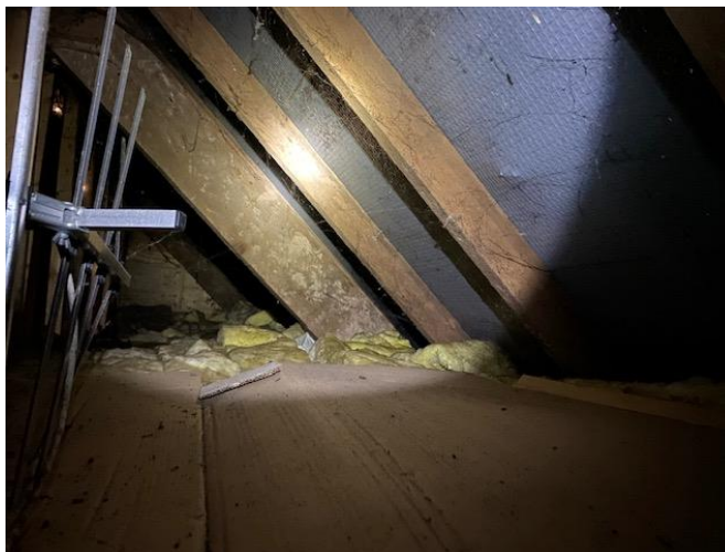
Photo 8. Loft space of dwelling
