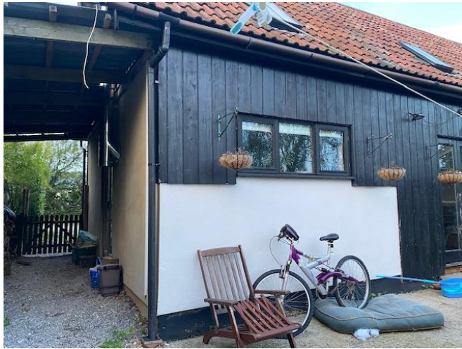
Photo 6. South west corner of dwelling
