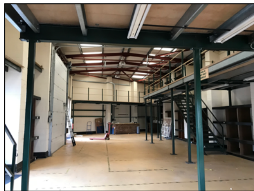
Figure 10 – internal space of the warehouse
