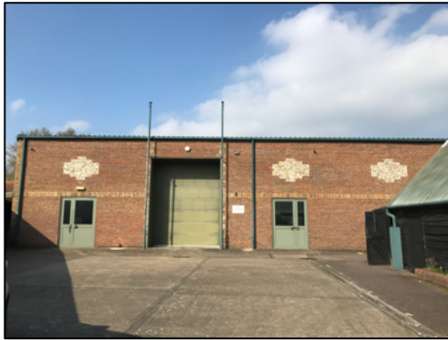
Figure 7 – the warehouse eastern elevation
