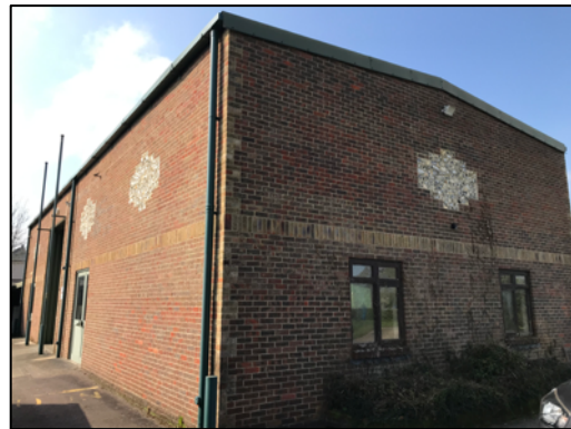
Figure 8 – the warehouse northern elevation
