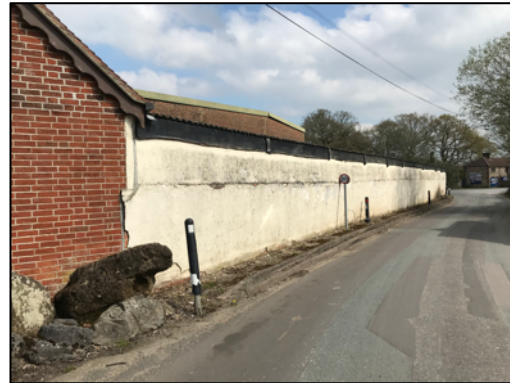
Figure 14 – the stables southern elevation
