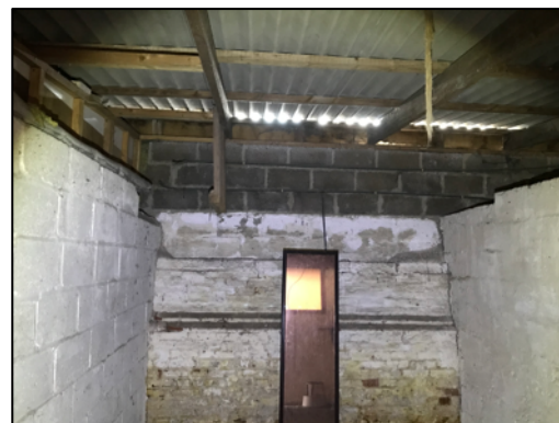
Figure 16 – internal view of the western stables
