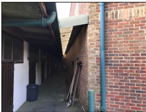
Figure 9 – covered shelter between buildings 2 and 3
