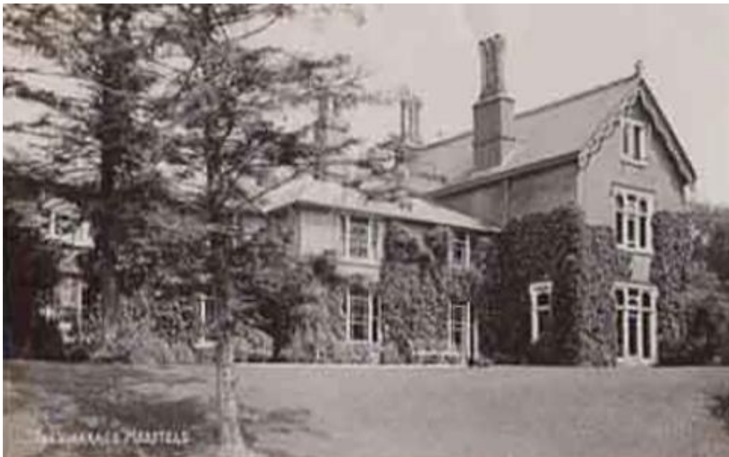
Side (Southwest) Elevation, shows the part of the rear wing which has been demolished
