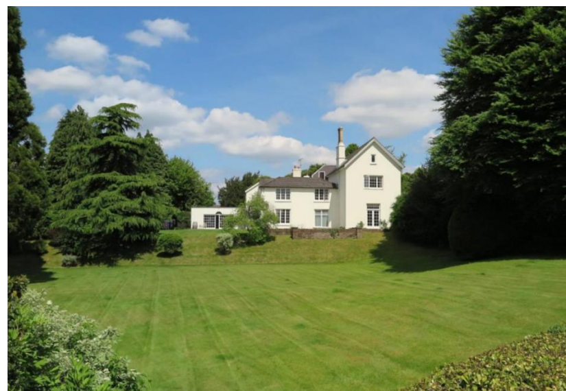
Side (Southwest) Elevation
