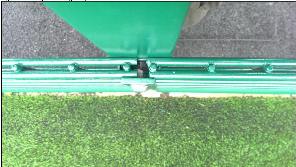
Figure 9: Image showing neoprene isolators
