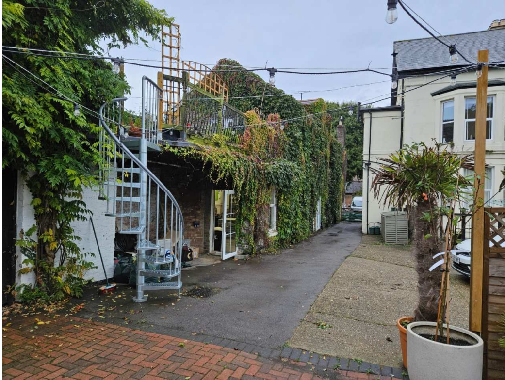
Fig 4 – View from the rear yard
