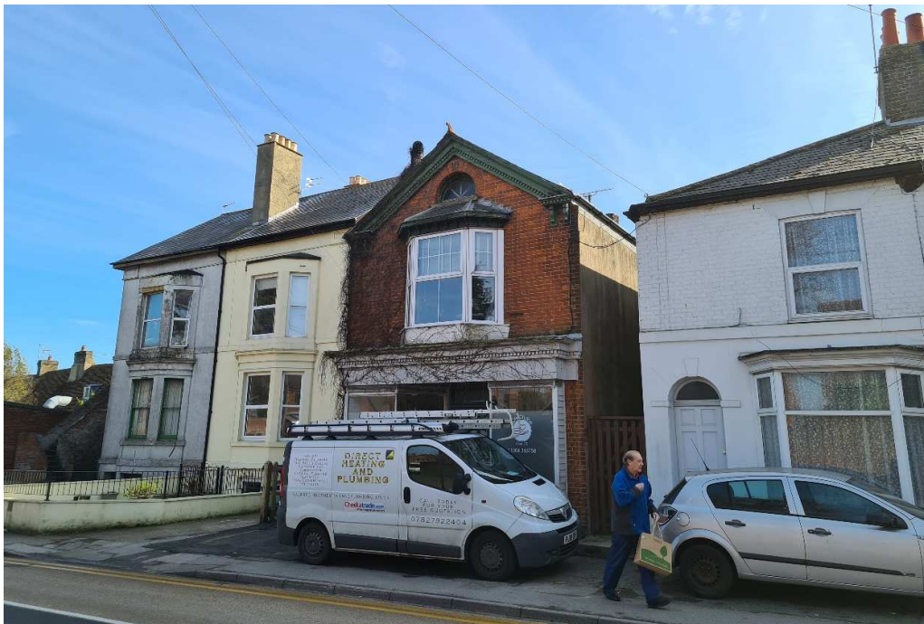
Fig 3.- Front view from London Road
