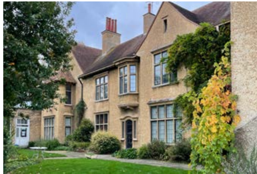
5 Rear entrance on the south east facing facade
