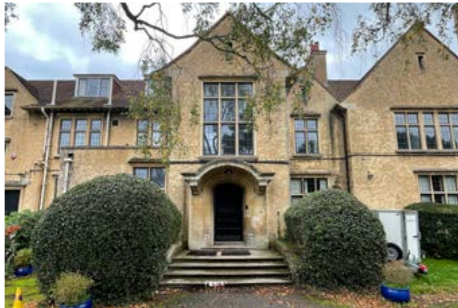
1 Existing main entrance with 6 steps up to the Finished Floor Level
