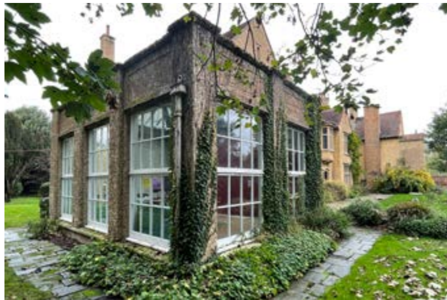
4 Southern corner of the building. Single storey Orangery
