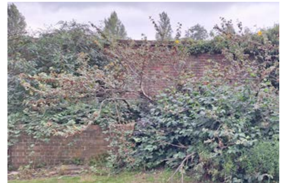
6 Planting and brick bund to the rear of the building
