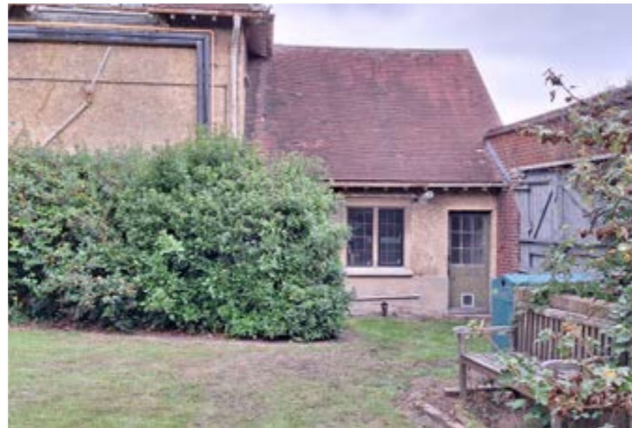
2 Rear entrance to workshop. Incoming gas meter box
