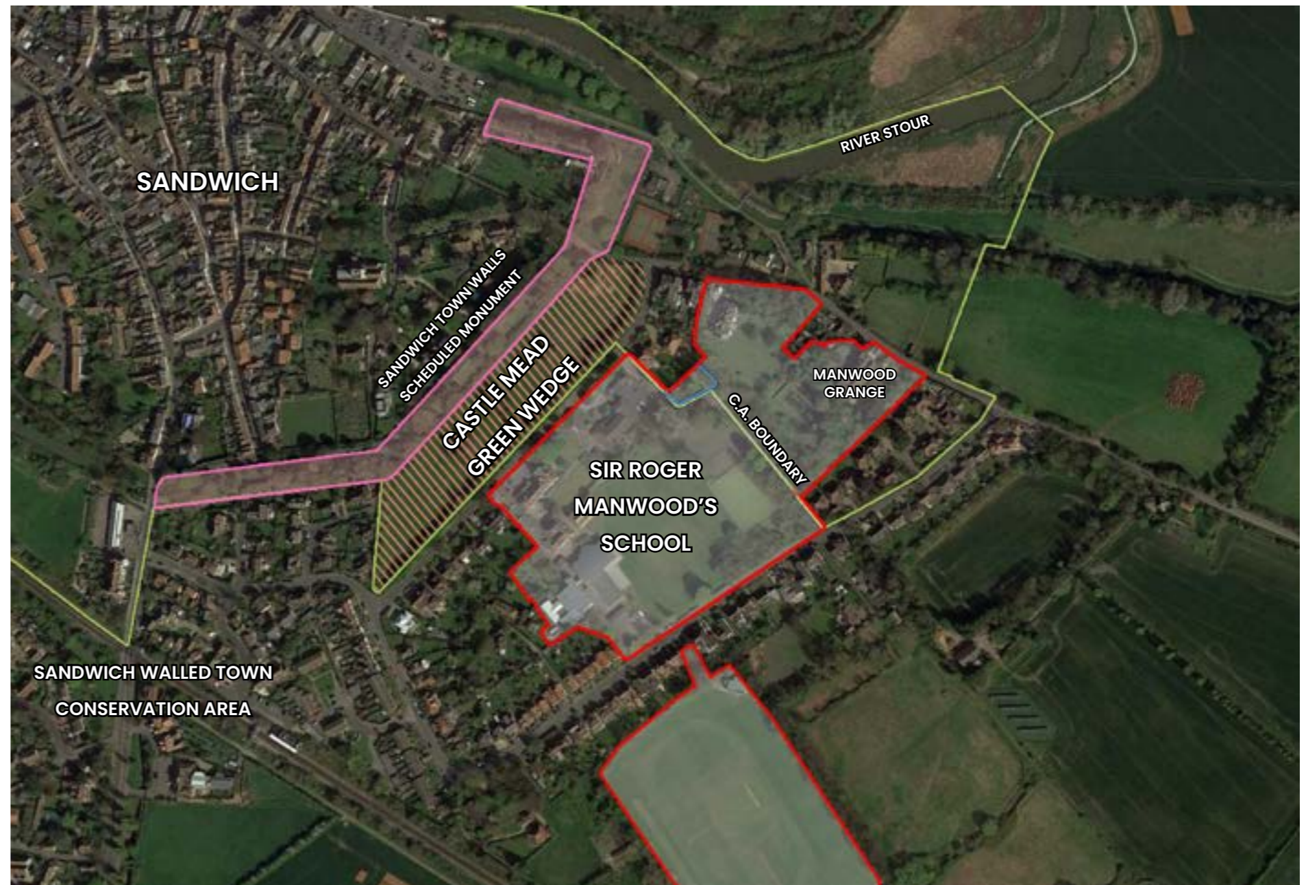
Aerial View showing the school's proximity to Scheduled Monument and overlap with the Conservation Area
