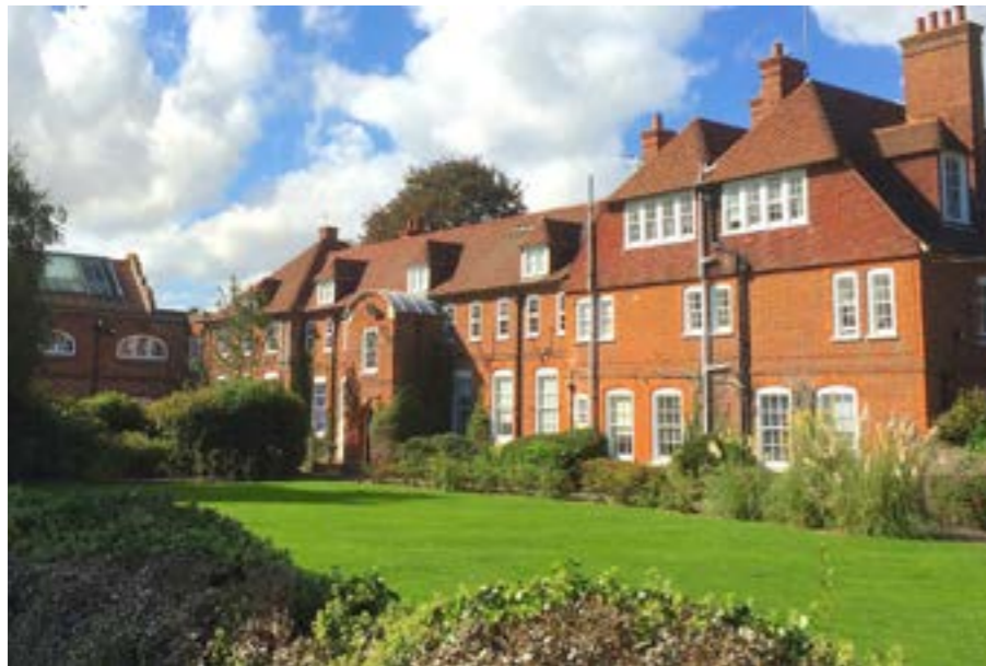
Existing school teaching block
