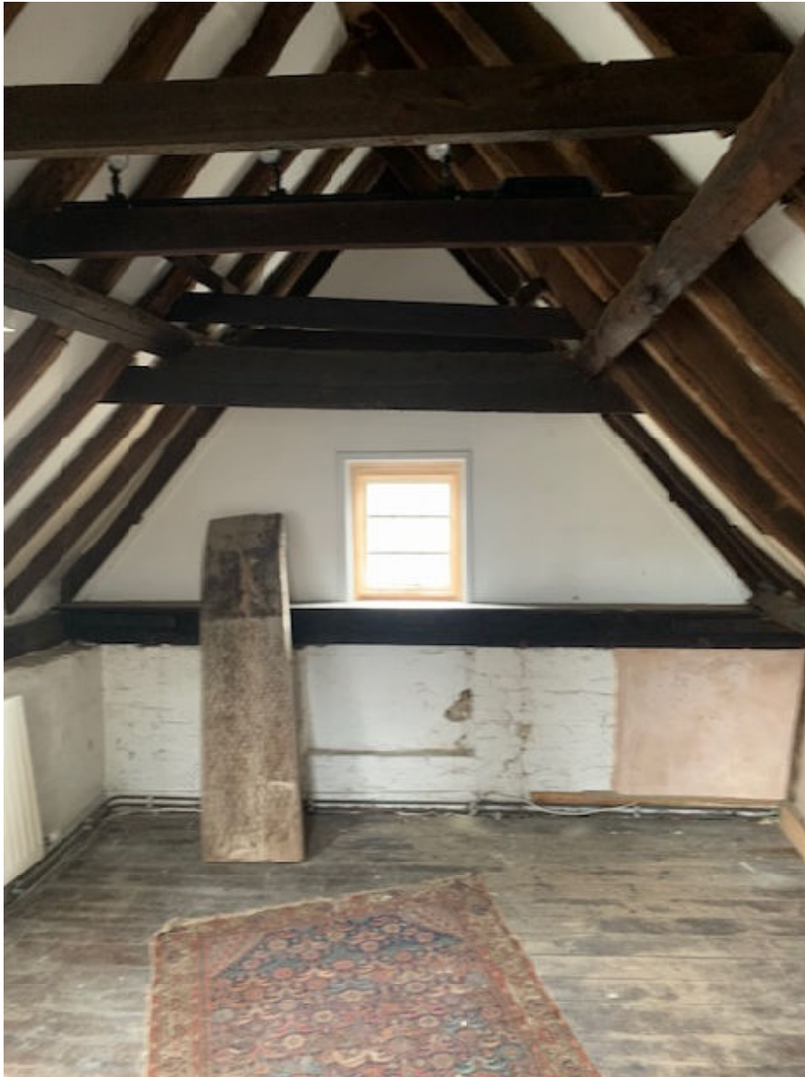
Internal View Showing Low Level Tie
