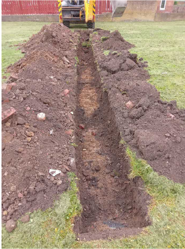
PLATE 1 – 28.04.22 TRIAL TRENCHING WITHIN AREA OF FORMER PUBLIC HOUSE TO CONFIRM ABSENCE OF RELIC FOUNDATIONS
