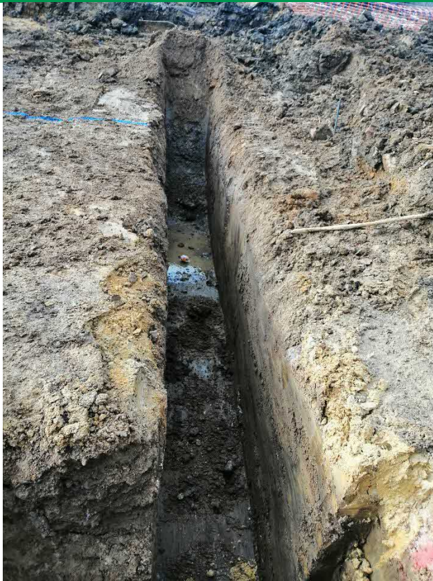
PLATE 2 – SHOWING FOUNDTION EXCAVATION IN CENTRAL SITE AREA
