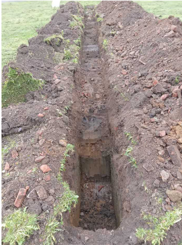
PLATE 2 – 28.04.22 TRIAL TRENCHING WITHIN AREA OF FORMER PUBLIC HOUSE TO CONFIRM THE ABSENCE OF RELIC FOUNDATIONS
