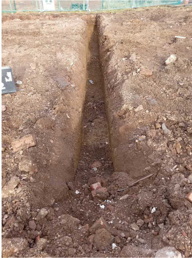
PLATE 5 – 03.02.23 INSPECTION OF TRIAL TRENCHES WITHIN SOUTHERN AREA OF THE SITE
