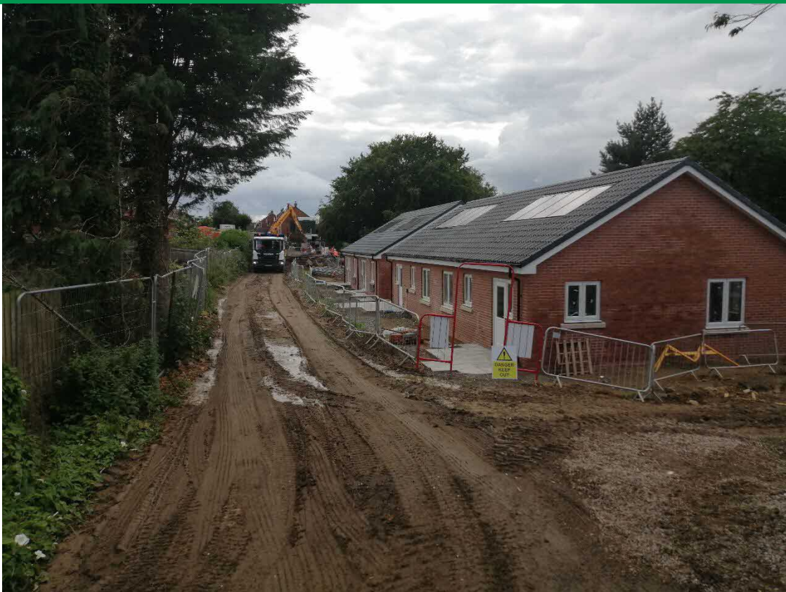
PLATE 8 - 15.08.23 HAUL ROAD TO REAR OF PLOTS 6-9
