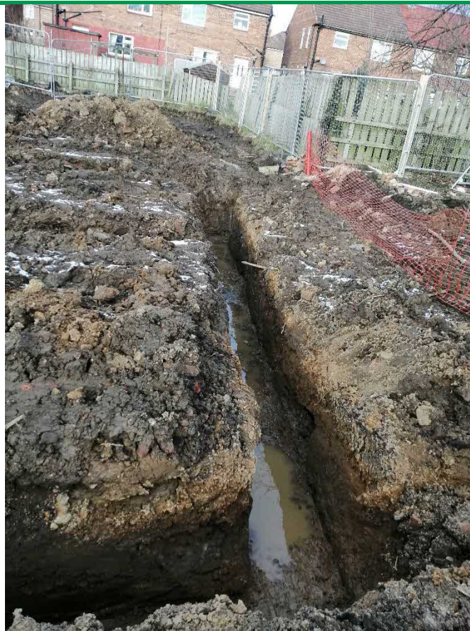
PLATE 4 – SHOWING FOUNDATION EXCAVATION IN NORTHERN SITE AREA
