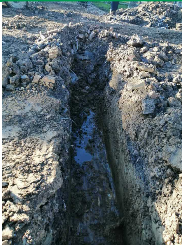
PLATE 8 – SHOWING TP201 WITH NATURAL CLAYS ENCOUNTERED AT BASE.
