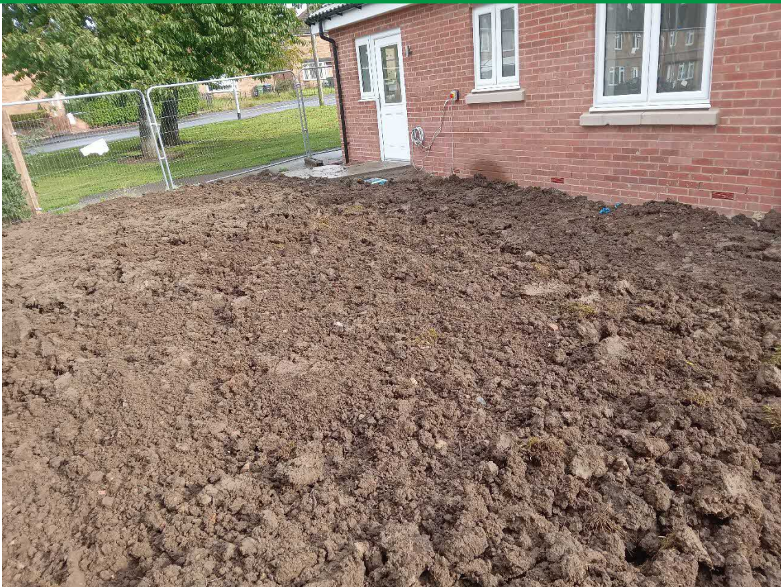
PLATE 2 – GENERAL PLACEMENT OF MATERIALS WITHIN PLOTS 1-2
