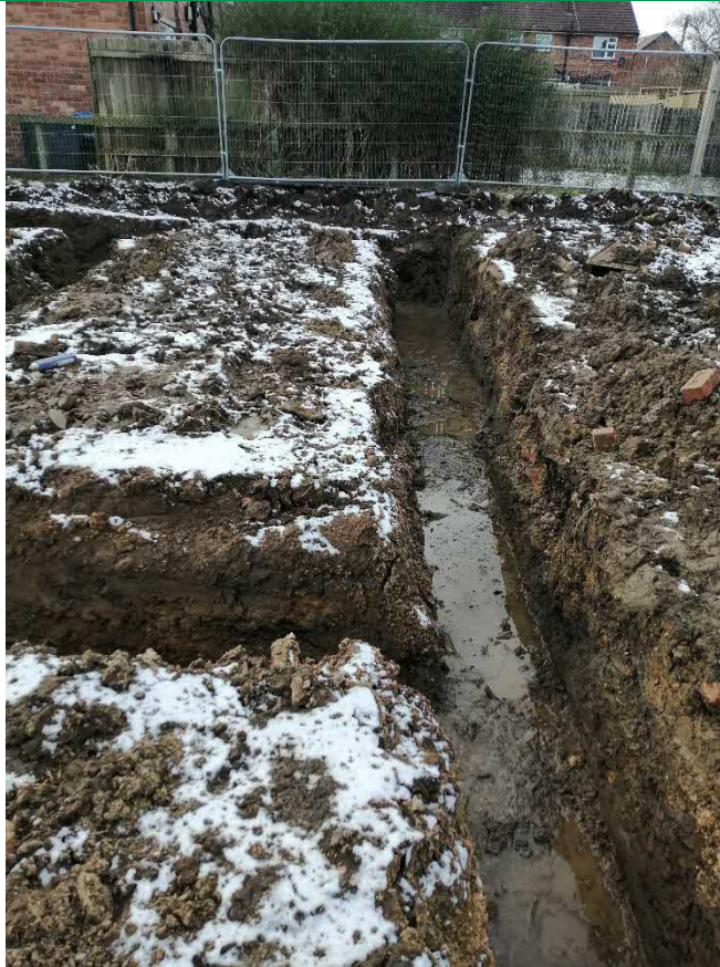
PLATE 5 – SHOWING FOUNDTION EXCAVATION IN NORTHERN SITE AREA
