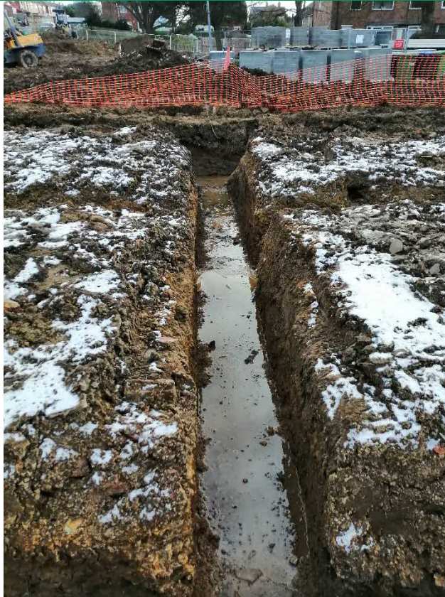
PLATE 6 – SHOWING FOUNDTION EXCAVATION IN NORTHERN SITE AREA
