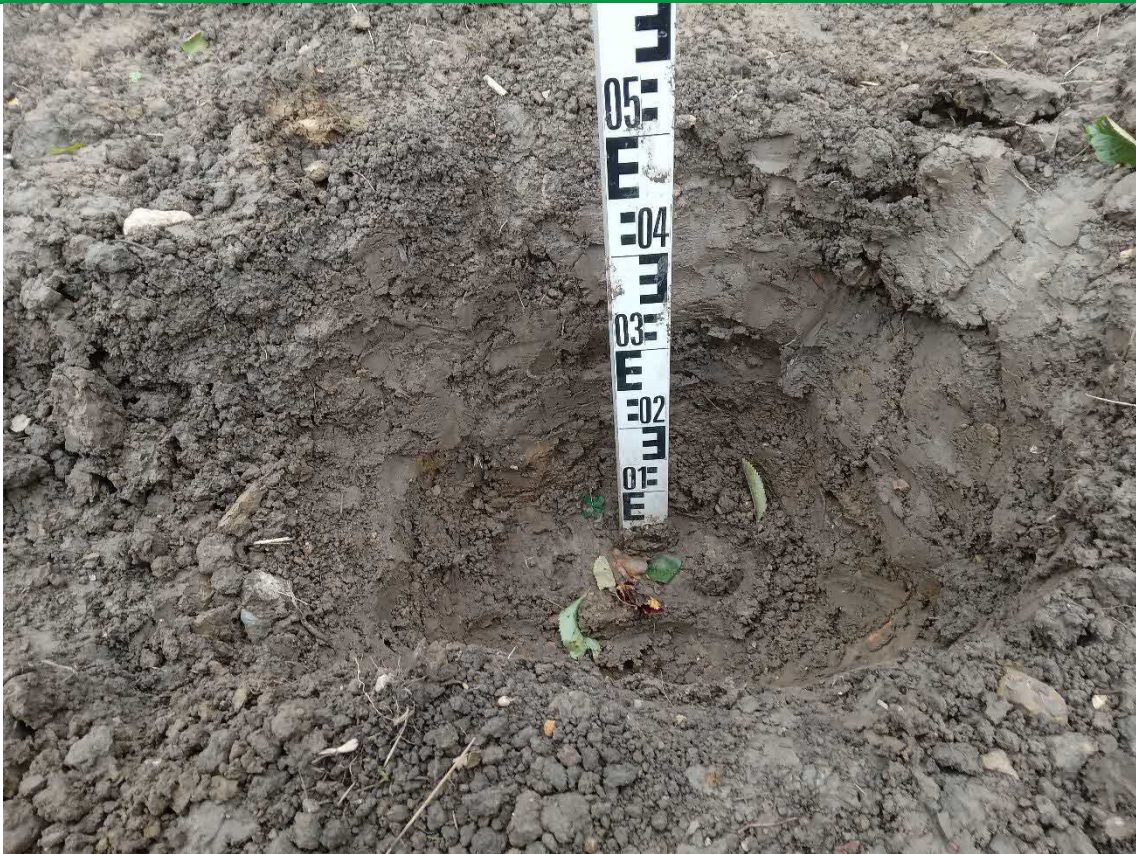
PLATE 3 – PLACED TOPSOIL MATERIALS AND DEPTH VALIDATION OF PLOT 4
