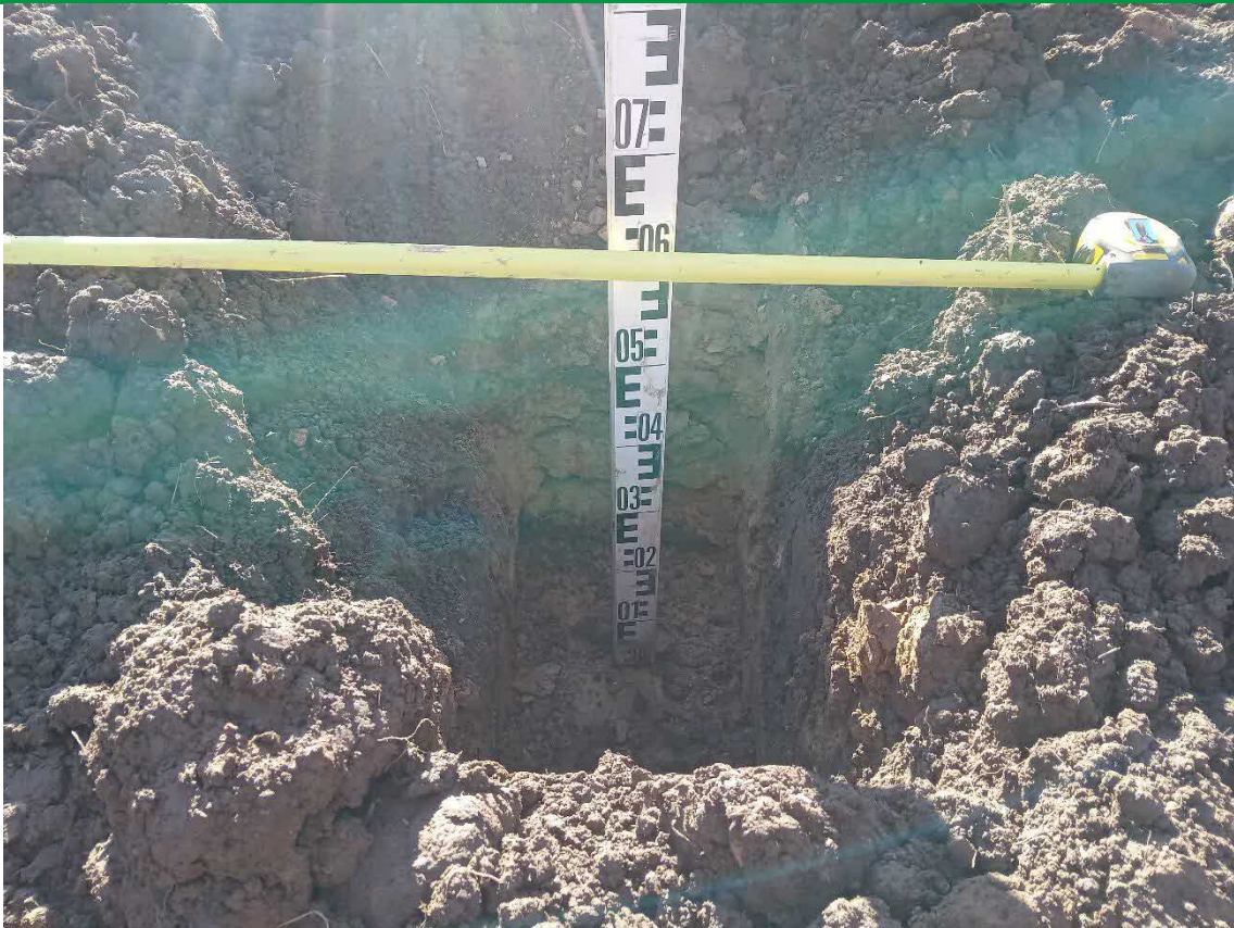
PLATE 3 – PLACED TOPSOIL MATERIALS AND DEPTH VALIDATION OF PLOT 9
