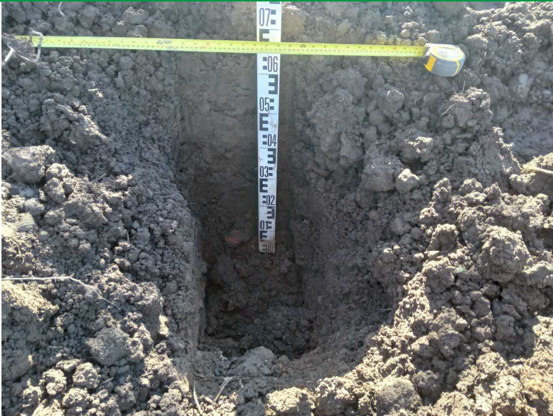
PLATE 7 – PLACED TOPSOIL MATERIALS AND DEPTH VALIDATION OF PLOT 15
