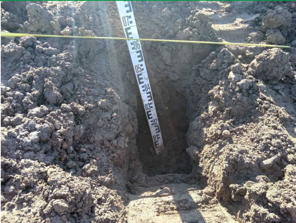
PLATE 5 – PLACED TOPSOIL MATERIALS AND DEPTH VALIDATION OF PLOT 13
