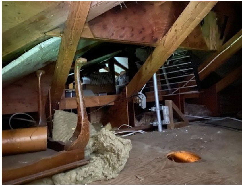
Loft view over north-east corner (2023)
