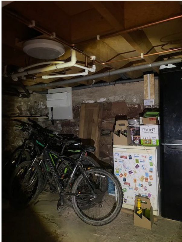
Inside cellar store room (2023)
