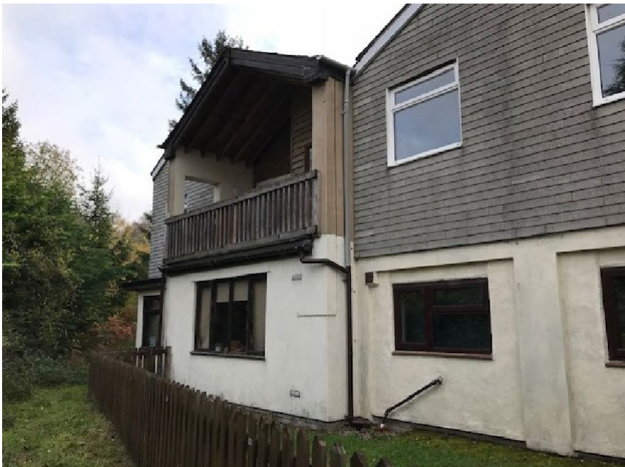
Front (north-west) elevation of Colebrooks – cladding to be altered (2018)
