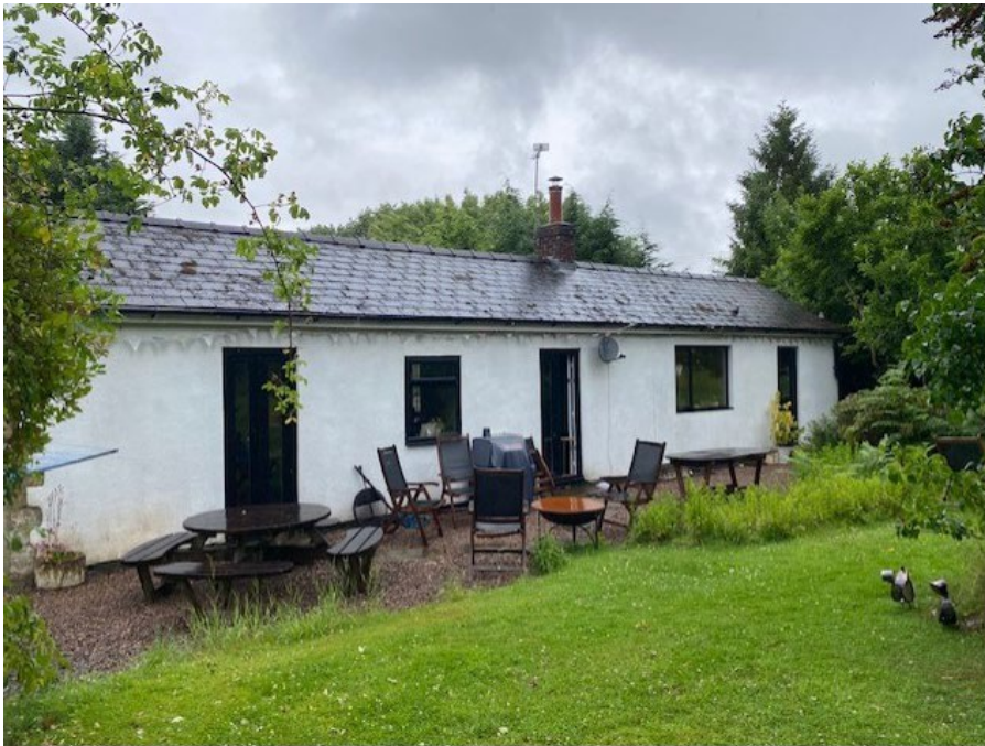
Rear (south-east) view of Colebrooks where single storey extension is proposed (2023)
