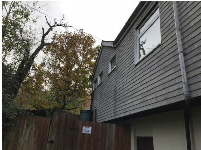
North-east side gable end (2018)
