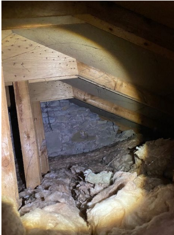
Loft view over south part of house (2023)
