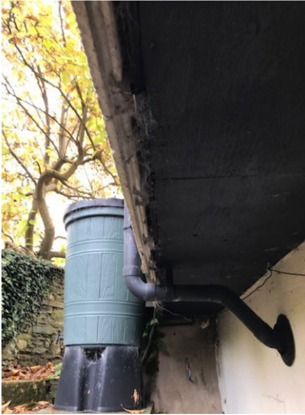
Under side of north-east gable (2018)
