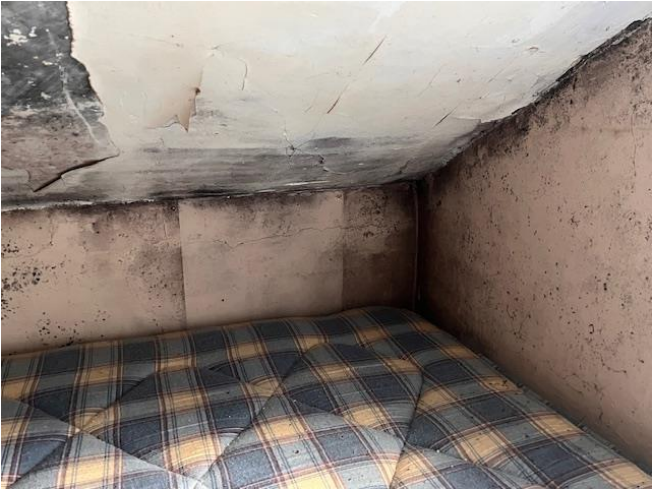
Some examples of damp and mould in the house:
