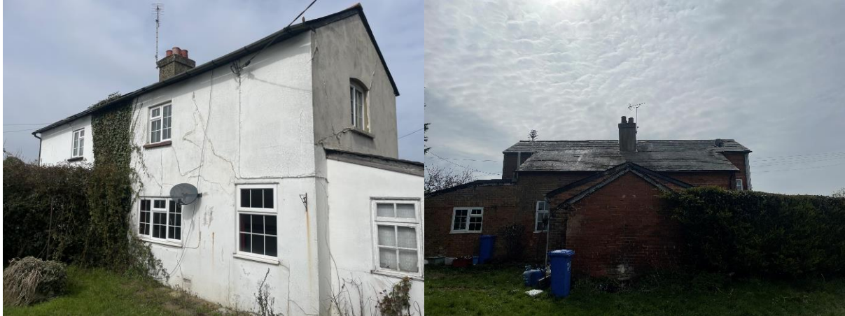
Existing 2no. semi-detached houses (front) Existing 2no. semi-detached houses (rear)
