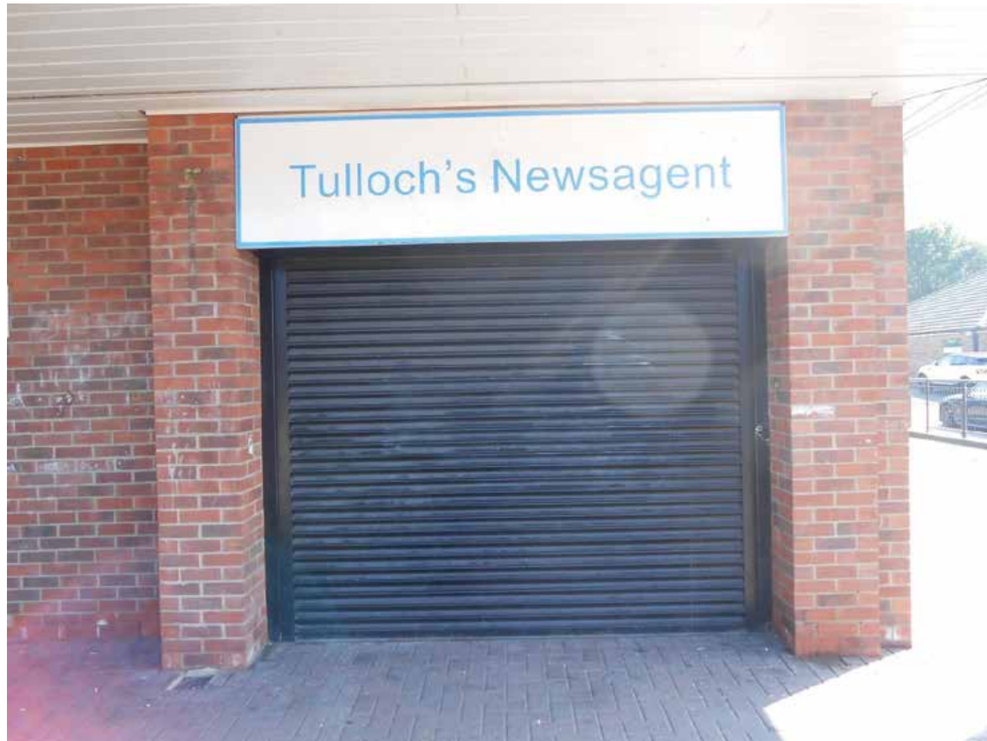
Existing Side view
