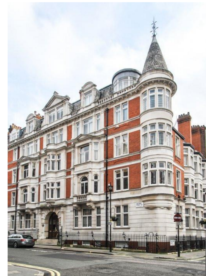
Bentinck Street Mansions 1-12 in the Edwardian style, located at the corner of Bentinck Street and Marylebone Lane.
