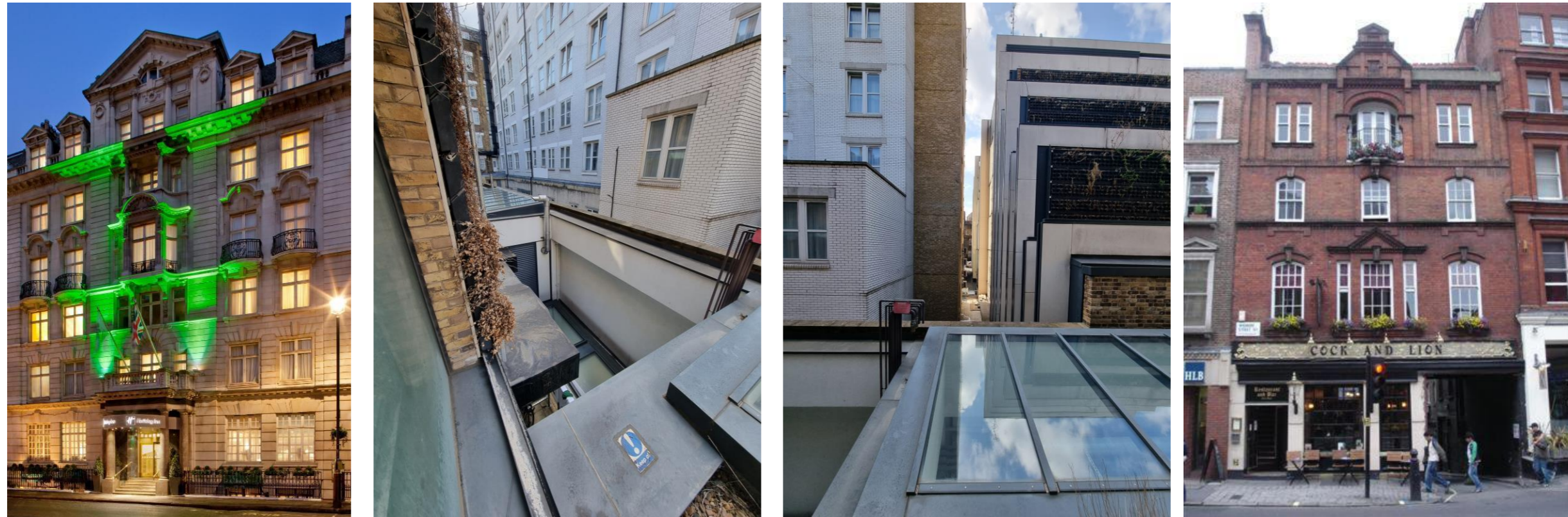
(Left Image) A hotel building (the Holiday Inn Hotel) fronting Welbeck Street is situated to the east of the site. (Left Middle) Rear of 18 Bentinck Street first floor roof looking at the rear of Holiday Inn which is predominantly white brick with little to no architectural features. (Right Middle) Rear of 18 Bentinck Street first floor roof looking at the Easleys Mews and the rear of the Cock and Lion public house. (Right) Frontage of the Cock and Lion public house with the Easleys Mews service route to the right-hand side of the main frontage.
