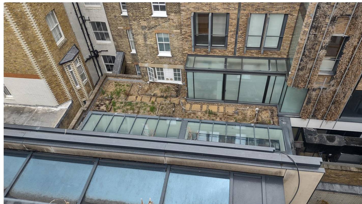
Site image from the 66 Wigmore Street fifth floor roof looking onto the 18 Bentinck Street First floor roof and existing contemporary glazed façade and rooflight. Left hand side is 1-12 Bentinck Street Mansions with gap between roof and 17 Bentinck Street.
