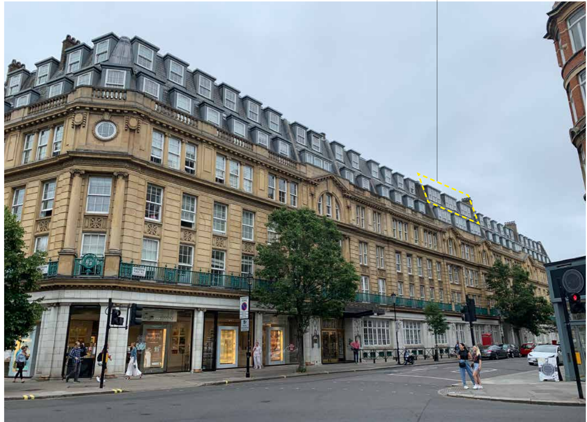
Above: An overall view of the block viewed from the junction of Chepstow Place with Westbourne Grove
