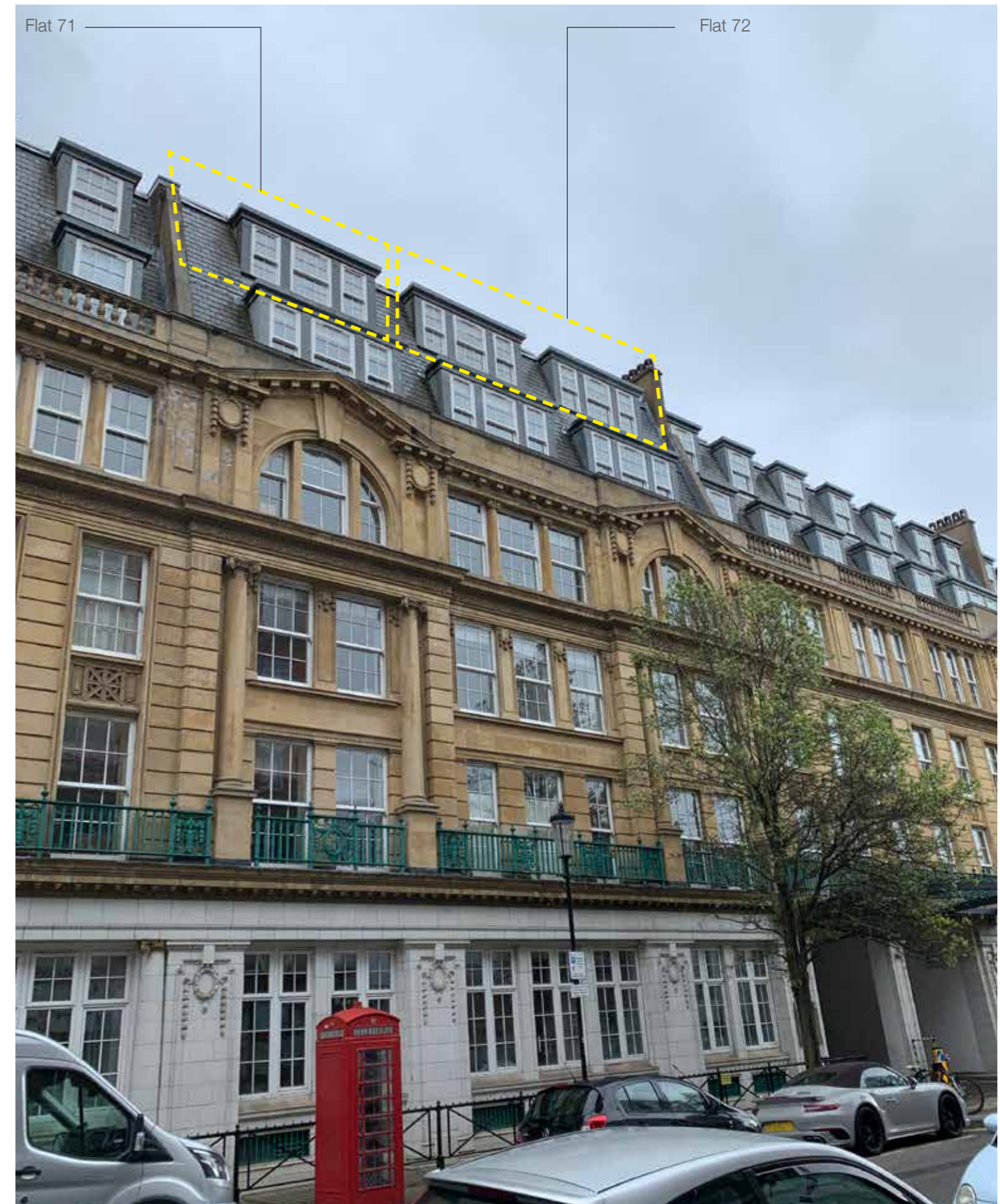
A view of Baynards House, from Chepstow Place - the street facing, west elevation
