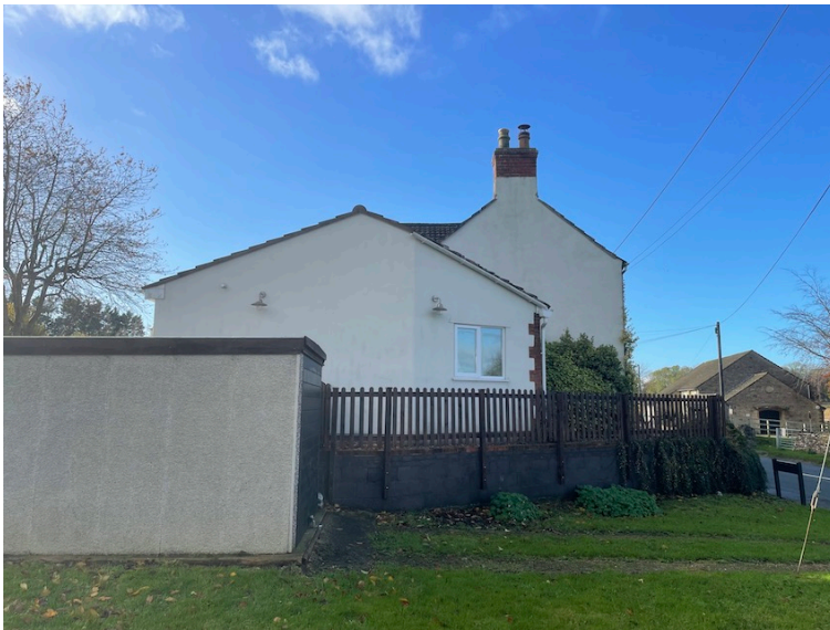
Existing end (north) elevation
