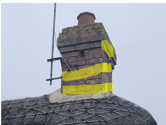
Photo 2: Front Chimney (south-east view)
