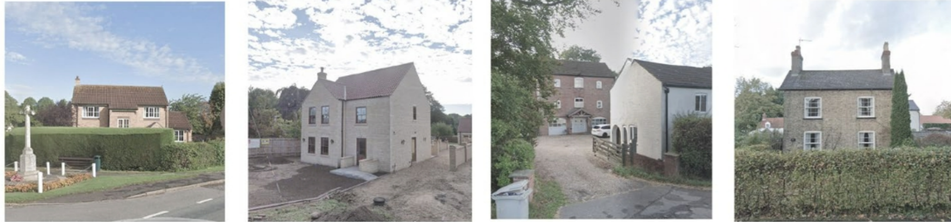
Houses within East Barkwith but not on Willingham Road, include stone, different brick types and rendering.
