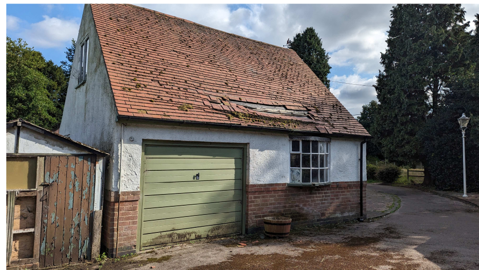
Fig 5 – Redmays Garage/ Stable building
