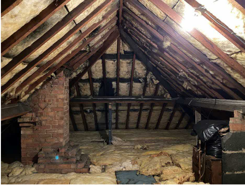
Loft void in B1
