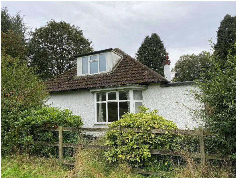
Eastern aspect of B1 showing loft extension dormer
