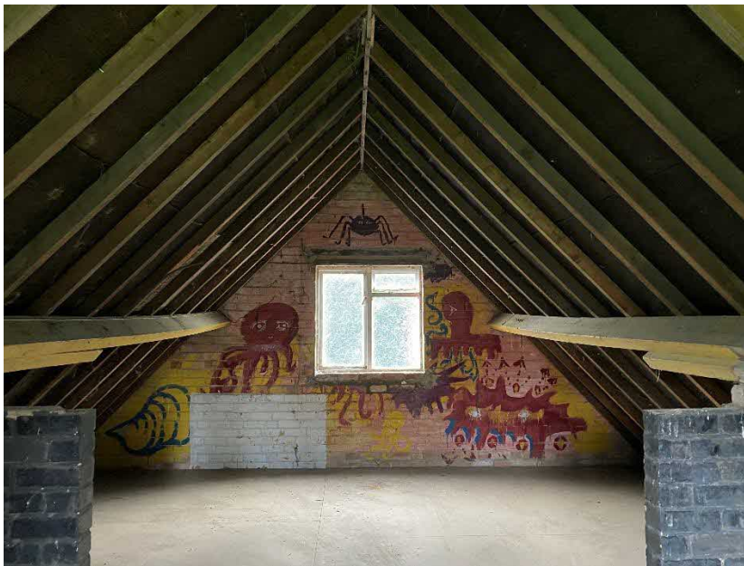
Upper floor level of B2
