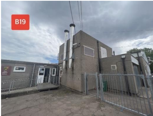
Photo 25 – Outside of B19
