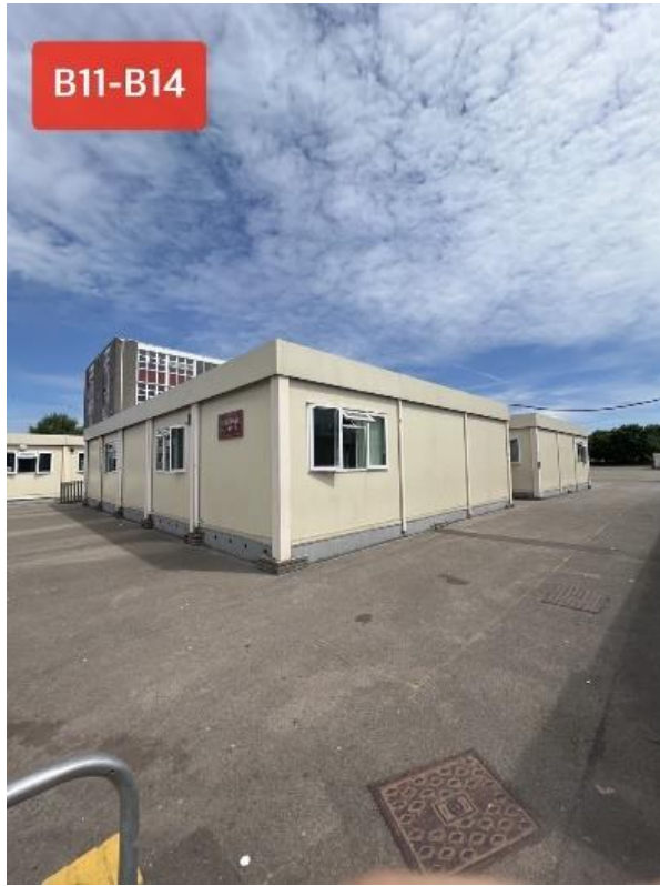
Photo 17 – B11 – B14 prefabricated buildings
