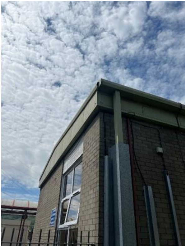
Photo 3 – TN2 – Building (B5) with house sparrow nest
