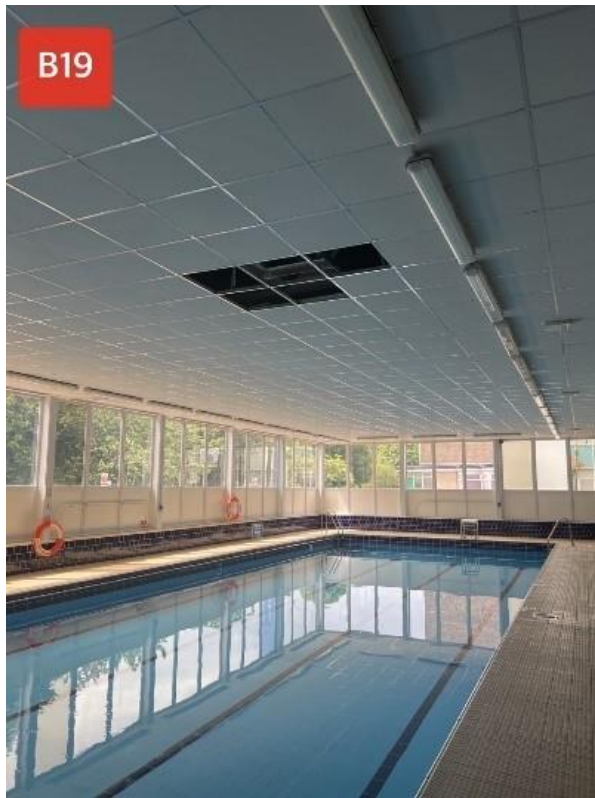
Photo 29 – Inside of B19
