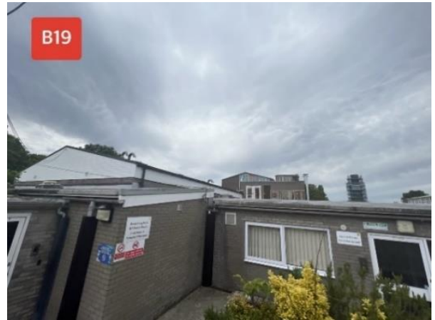
Photo 26 – Outside of B19
