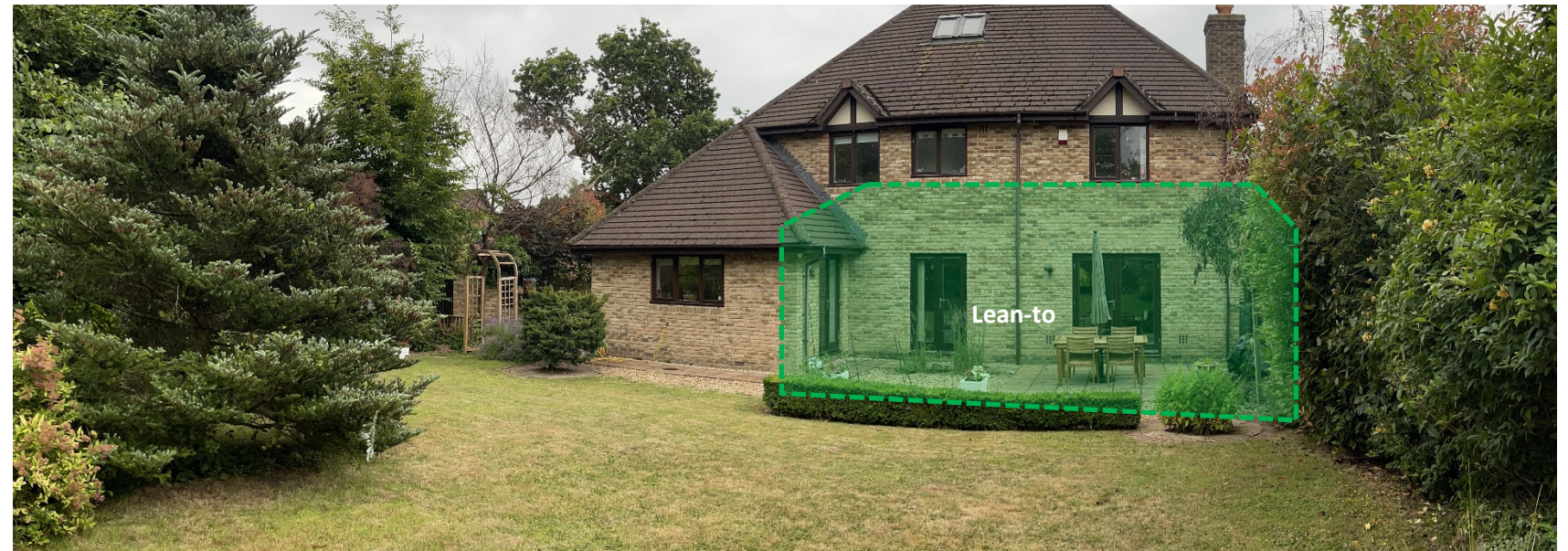
Kitchen/diner lean-to extension on patio area
