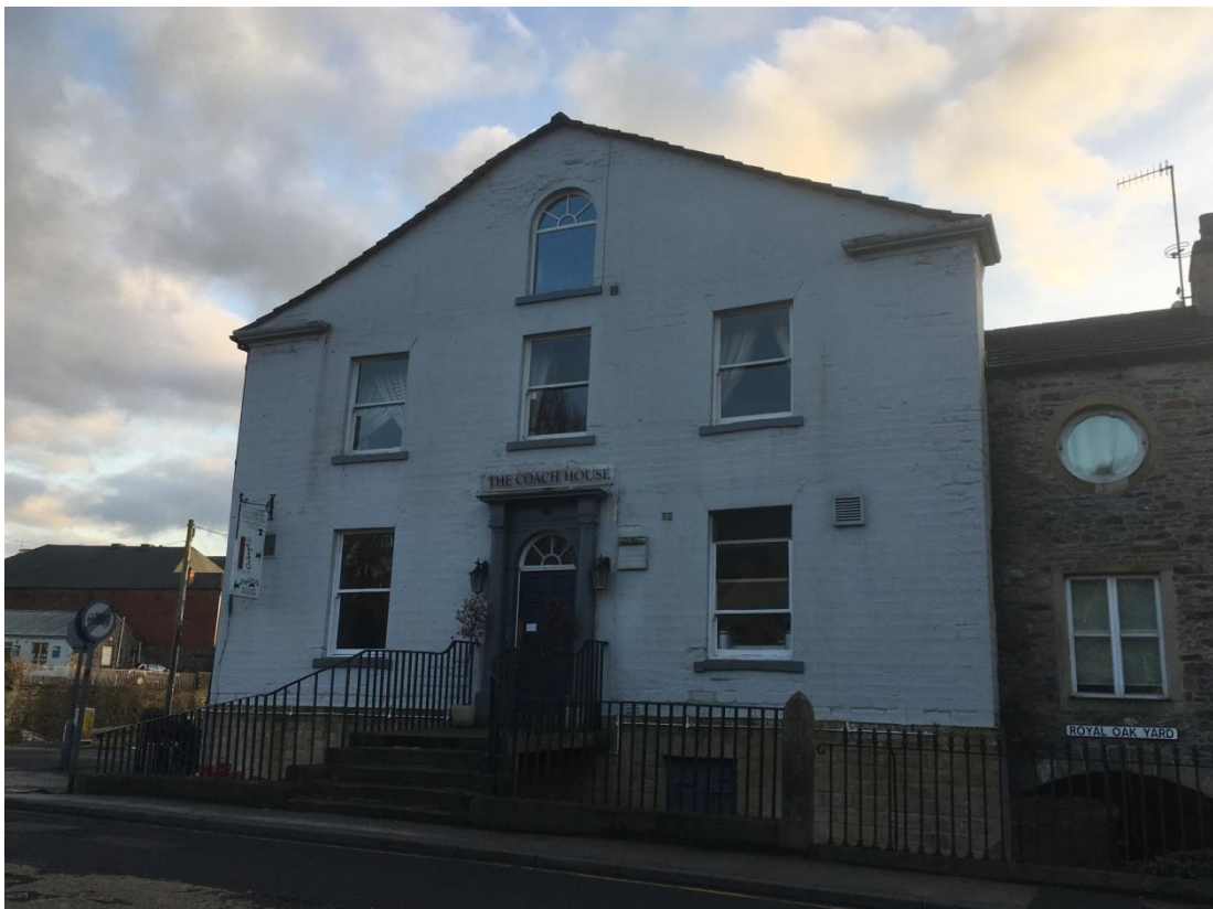
Figure 7: Gable end elevation facing on to Raikes Road, showing the grid formation of the openings typical of the Georgian period and the, presumed, original sash windows. Note the building set back and up from the roadside
