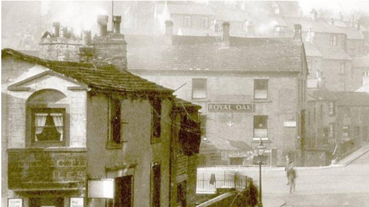
Figure 5: Picture marked as taken in 1875 (source: Old Skipton Pics – Facebook) showing the original 4no chimney stacks and no rooflights
