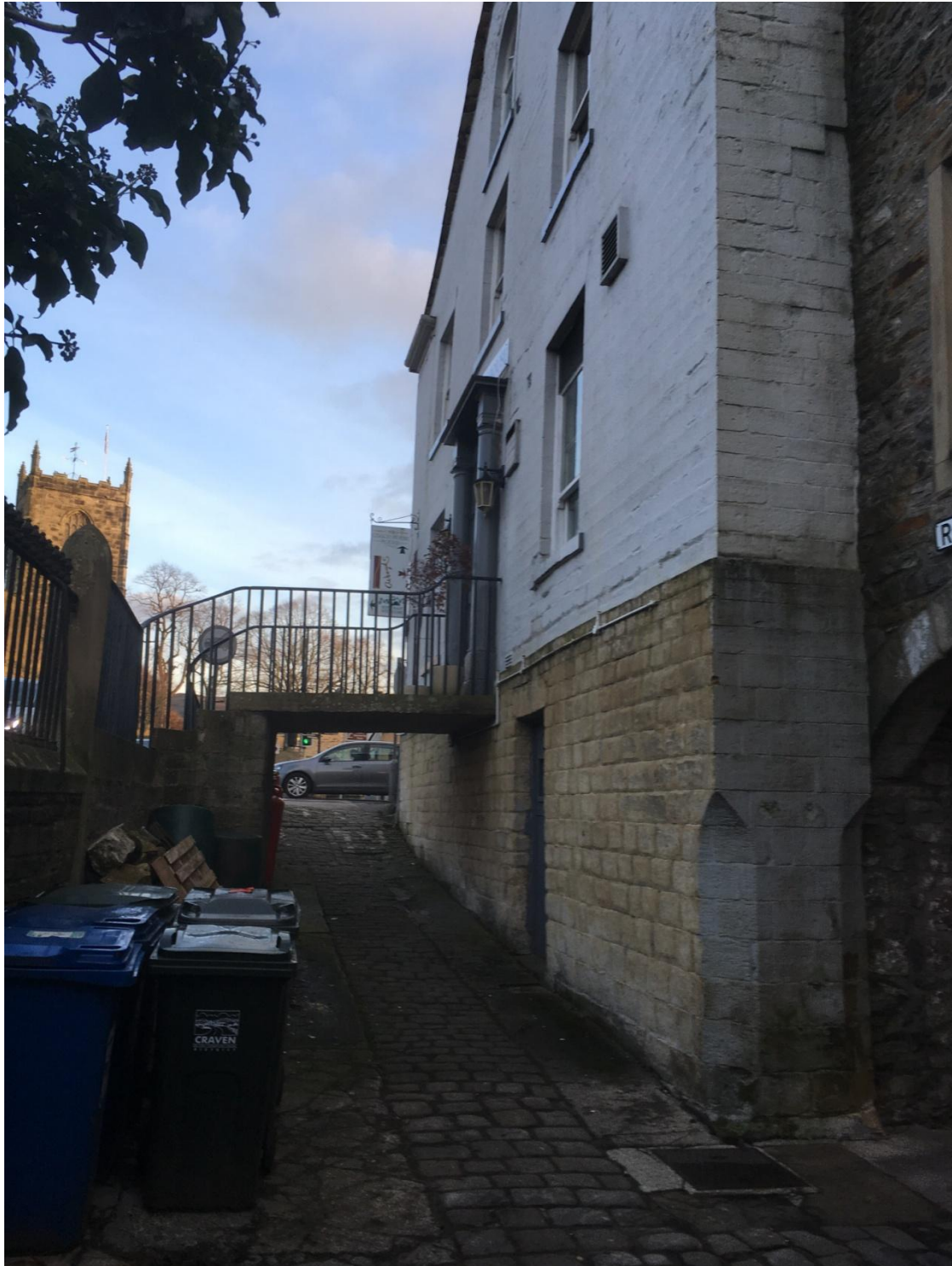
Figure 10: Building set back and up from roadside to enable horse and carriage entrance from Water Street. Access to the first floor is via stone steps and stone walkway. Note chamfered stone detailing at base of elevation by the archway
