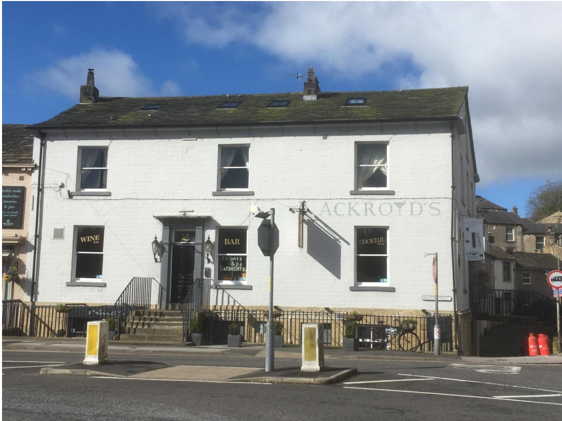
Figure 6: Elevation facing on to Water Street showing the grid formation of the openings typical of the Georgian period. Note the 2no chimney stacks and 4no roof lights.
