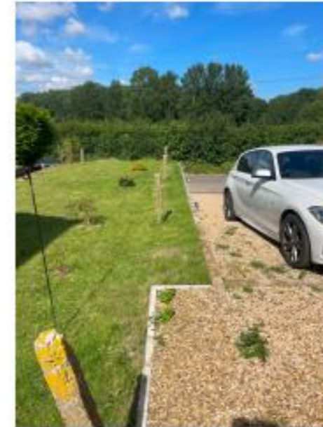
Gabion/ Sleeper retaining wall proposed to retain dividing boundary line to left hand side of kerb edging in above image
