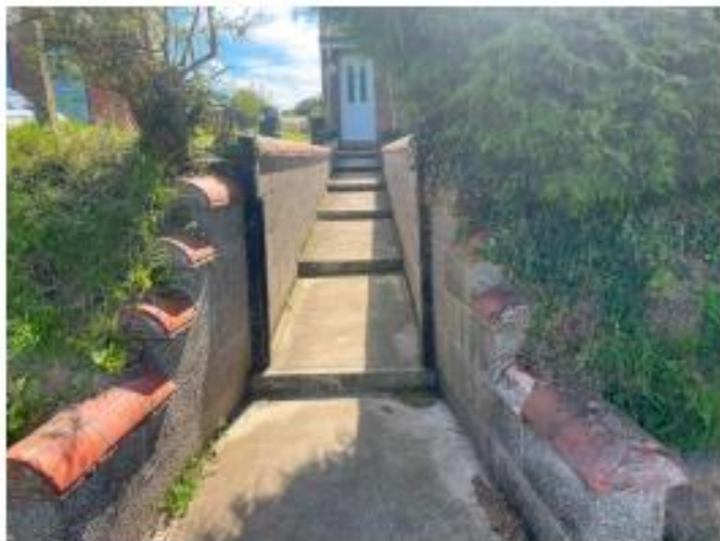
Left hand side retaining wall and concrete steps to be removed.
