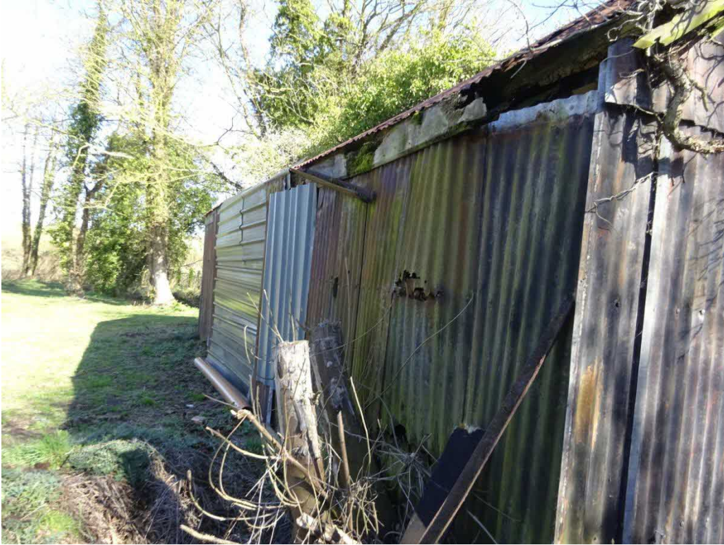
Photo 14. View of the large gap between the sarking and metal cladding of the building
