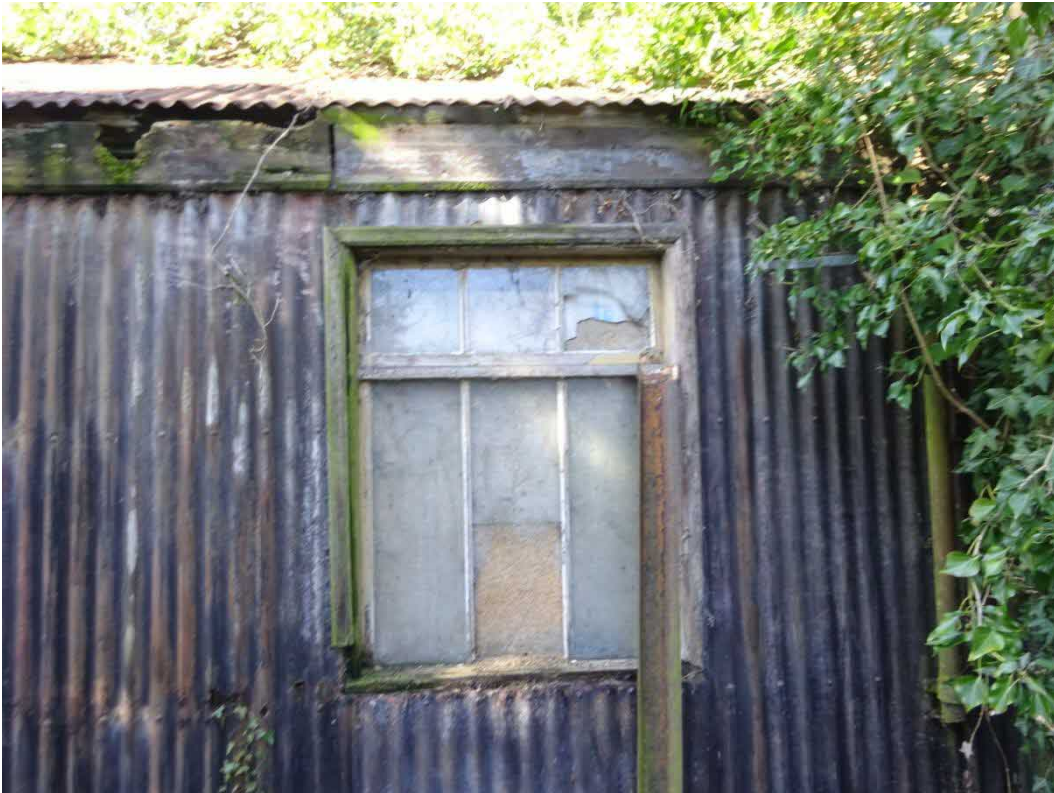
Photo 16. Example of the rotting fascia boards of the building
