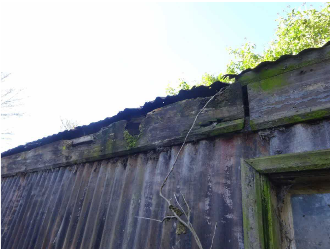
Photo 16. Example of the rotting fascia boards of the building
