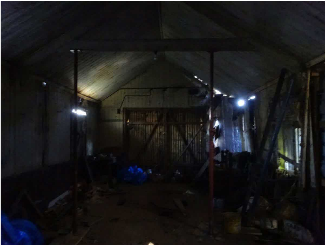
Photo 12. The metal supports installed to stabilise the building
