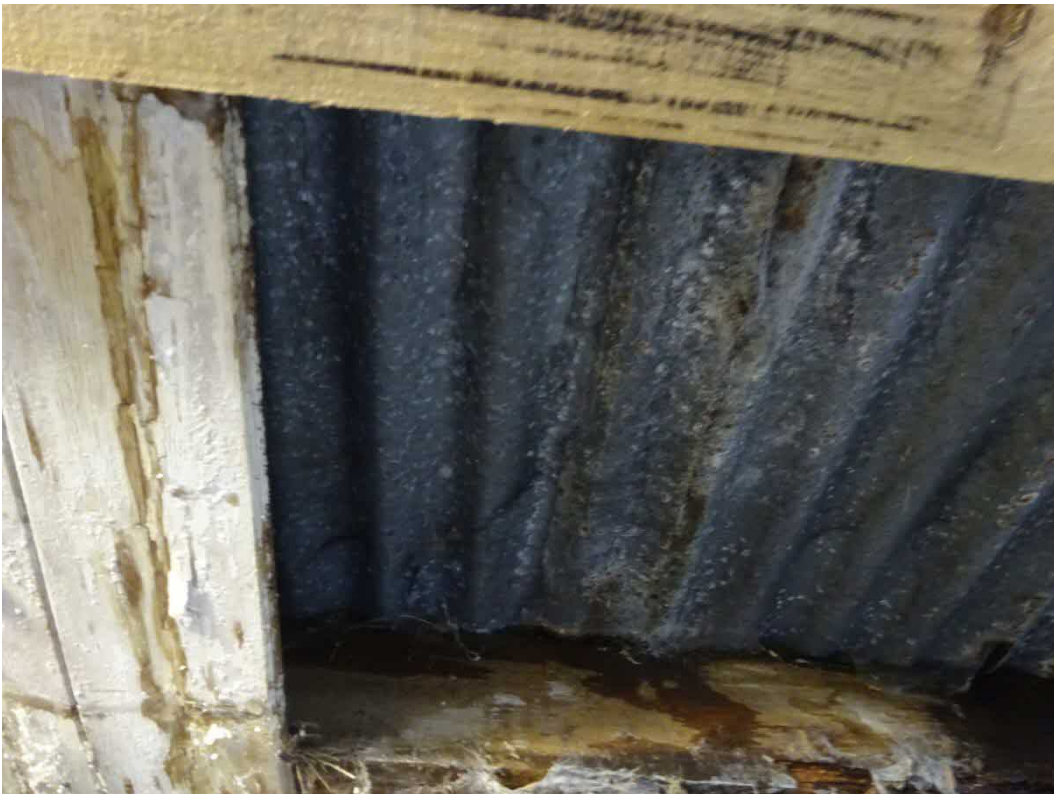
Photo 14. View of the large gap between the sarking and metal cladding of the building
