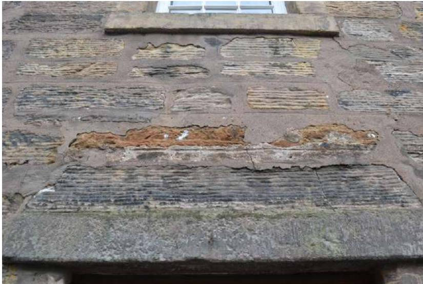
6. Cement mortar pointing on south elevation
