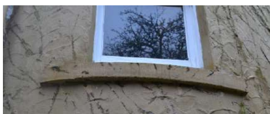
Concrete cill on turret extension indicating later construction
