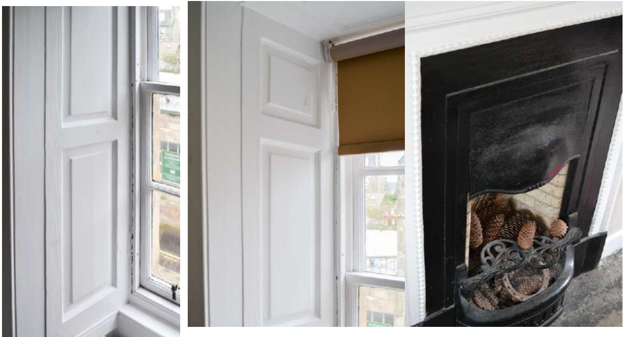
22. Wood Shutters & Cast Iron Fireplace, East Bedroom
