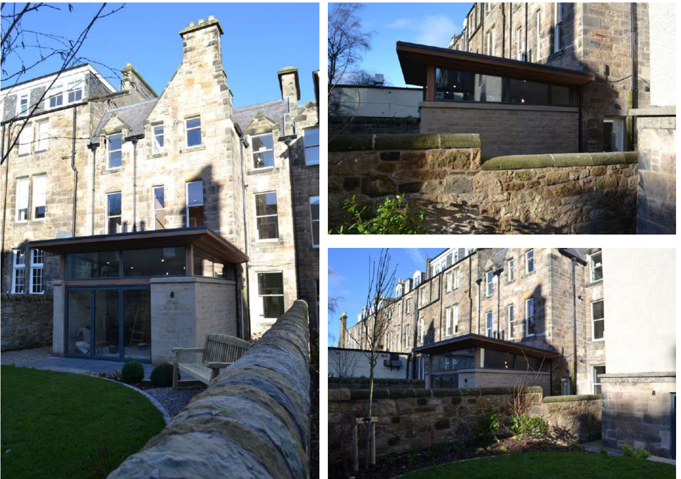
74. Rear extension to 30 The Scores in St Andrews by Andrew Black Design using a similar material palette as the proposal for 23 Market Street
