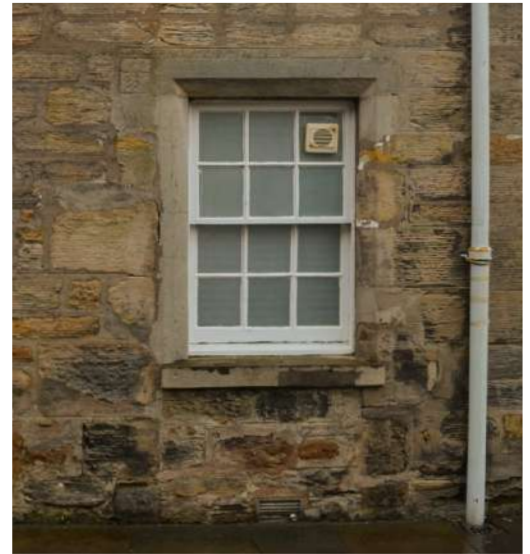
7. Bottom right window with altered concrete jamb, stone infill, obscured glazing & fan, detail
