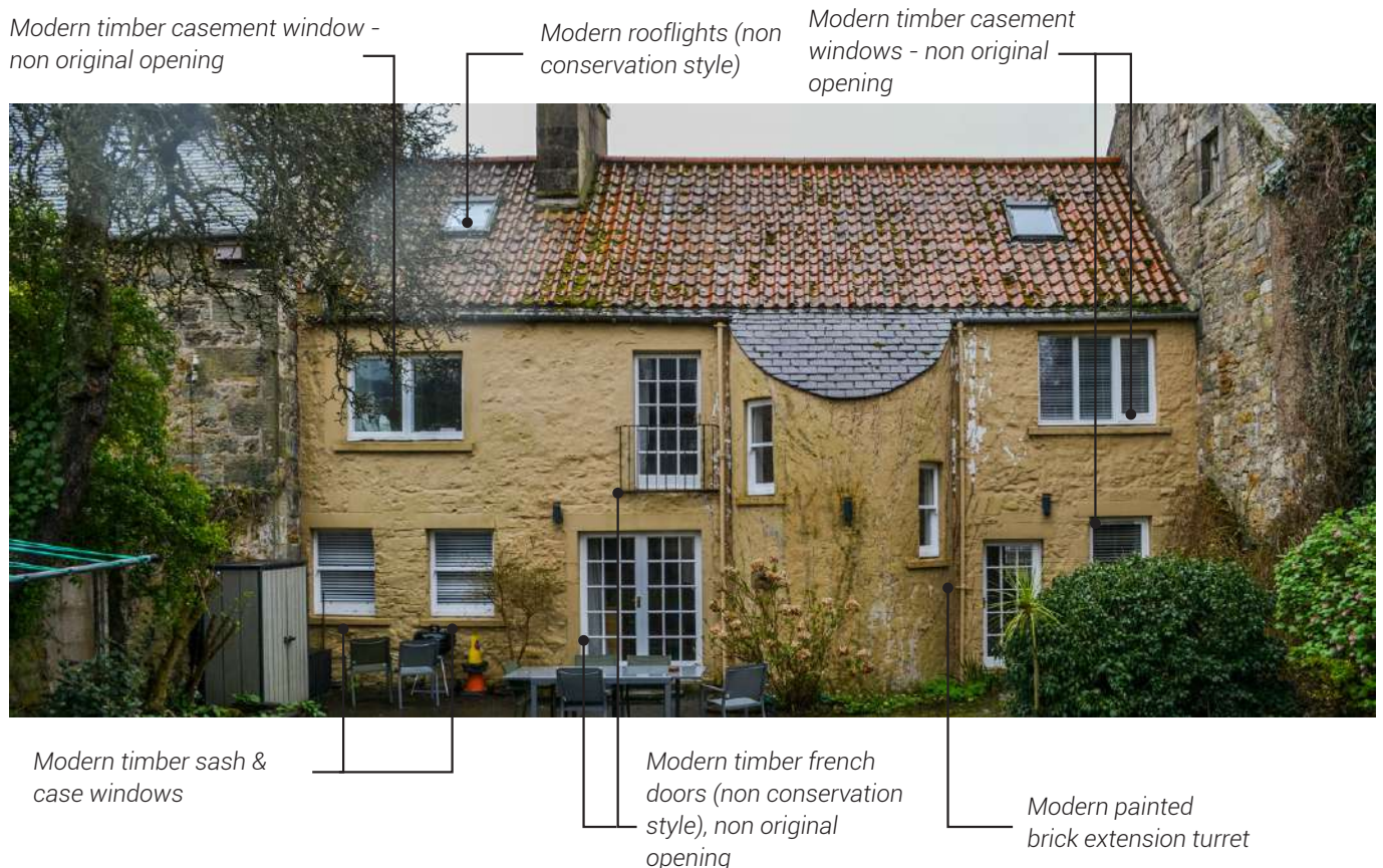
8. North Elevation - Garden - Observed alterations
