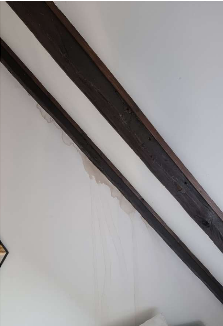
32. Roof Fabric - Details showing obvious signs of movement in the roof structure and the poor quality of the the roof insulation. The signs of water ingress on the gable wall also demonstrate the roof's need of urgent repair.
