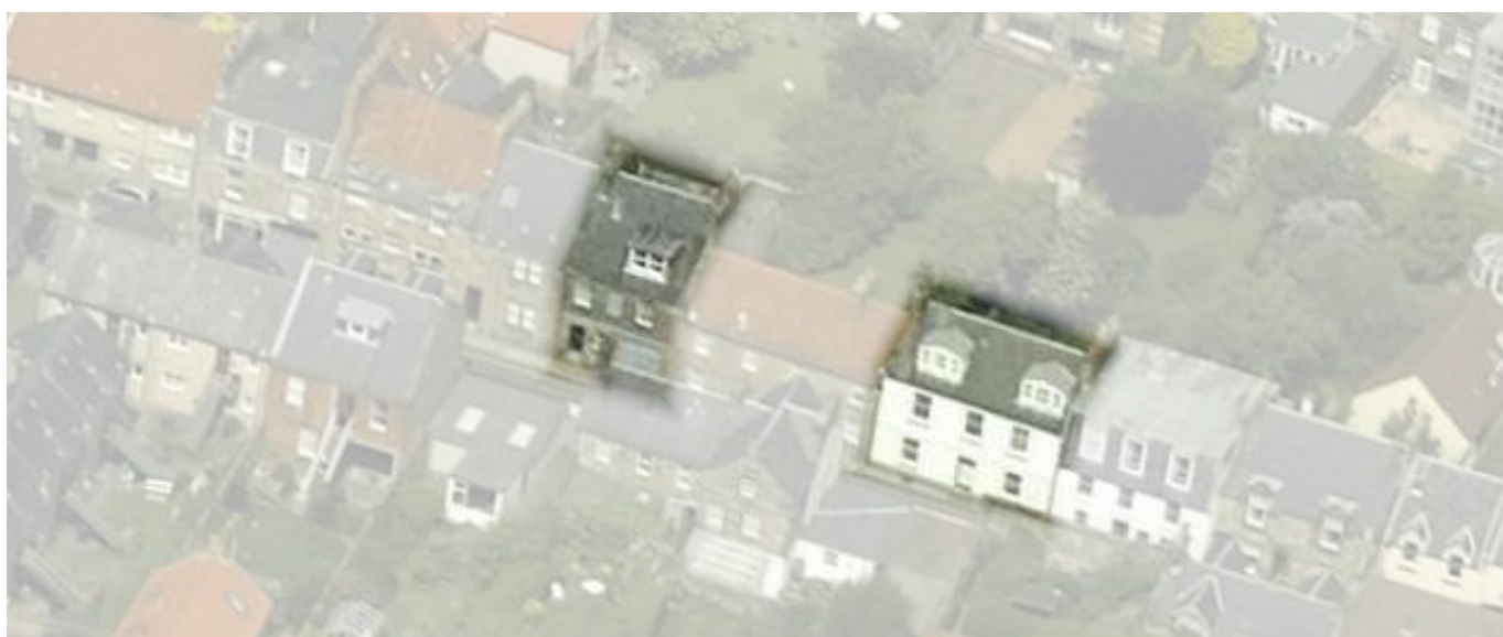
45. In 2006, 21 & 25 Market Street, are showing much bigger dormers. Other dormers have appeared on the street.
