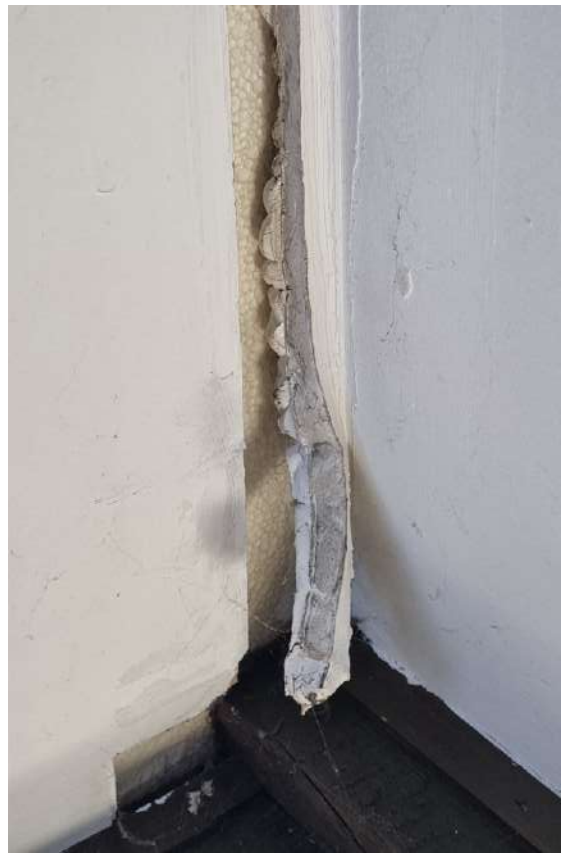
32. Roof Fabric - Details showing obvious signs of movement in the roof structure and the poor quality of the the roof insulation. The signs of water ingress on the gable wall also demonstrate the roof's need of urgent repair.
