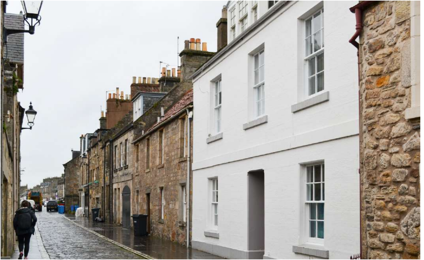
50. Existing Elevation Viewed from the East
