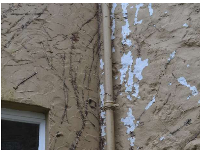
Texture difference between painted stone and painted brick of the extension
