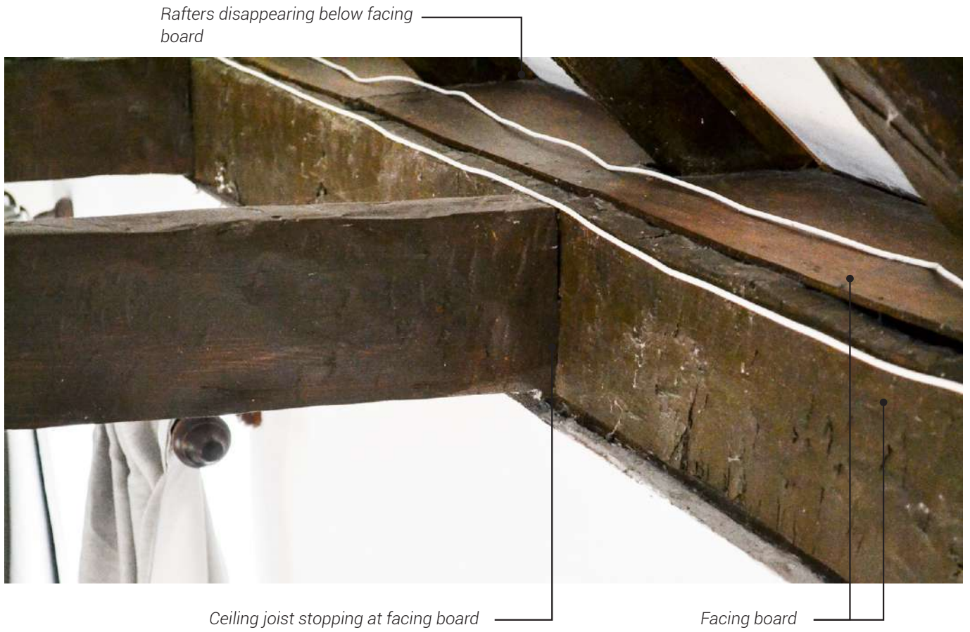
28. Existing Roof Structure
