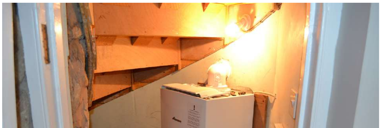
19. Underneath of staircase - modern plywood construction
