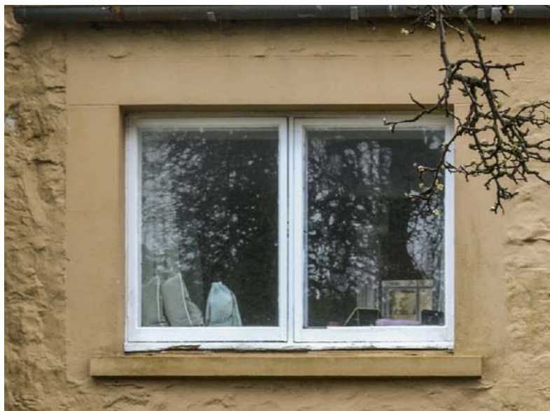
9. Modern timber casement window and french doors with concrete lintel, cill and surrounds
