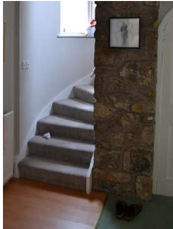
16. Opening in original stone wall to create stairs
