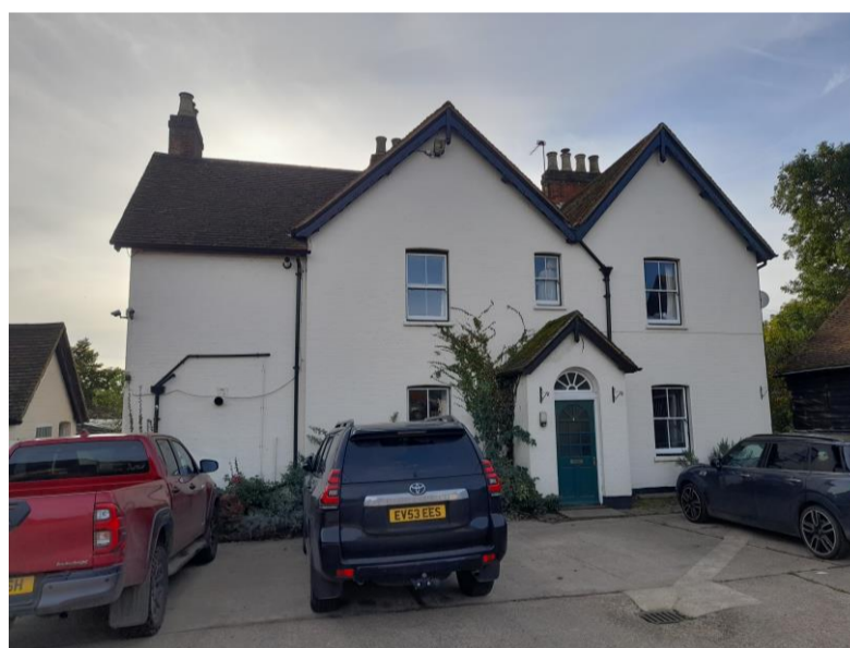
Photograph 19 Front elevation of Grade II listed Pursley Farmhouse
