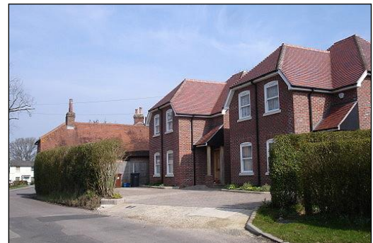
New development with unresolved threshold to street. Pound Lane
