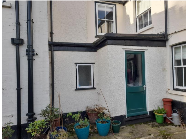
Photograph 4 View of rear elevation showing flat roof to single storey extension
