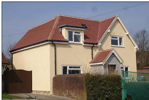
Bulky roof form resulting in visually discordant appearance. Harris Lane
